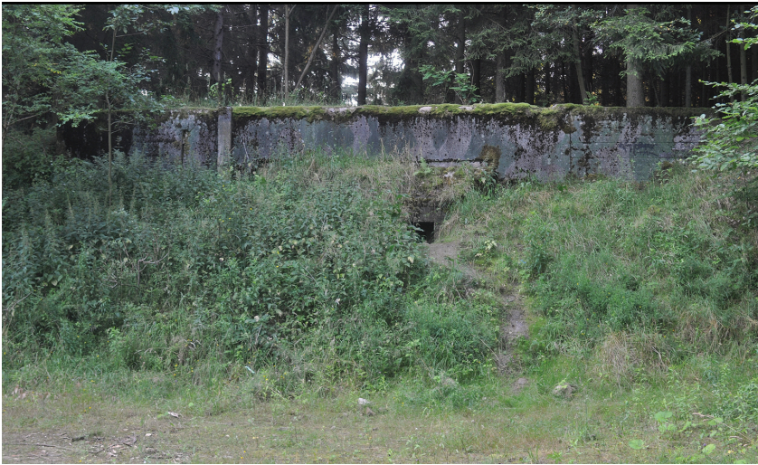
Figure 1. Partly blocked entrance to the bunker system. In the background, pine-spruce forest overgrowing the hillock built to camouflage the structure. Photo taken on 17.07.2014 (Wojciech Stephan).
