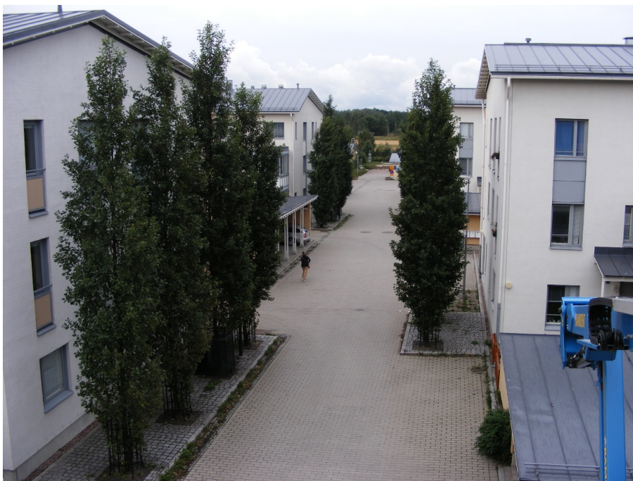
Figure 2. The Alnus site photographed from boom lift in August 2010; view is from north towards south. Planting pockets with their granite unit pavers were arranged along the street paved with concrete unit pavers.
