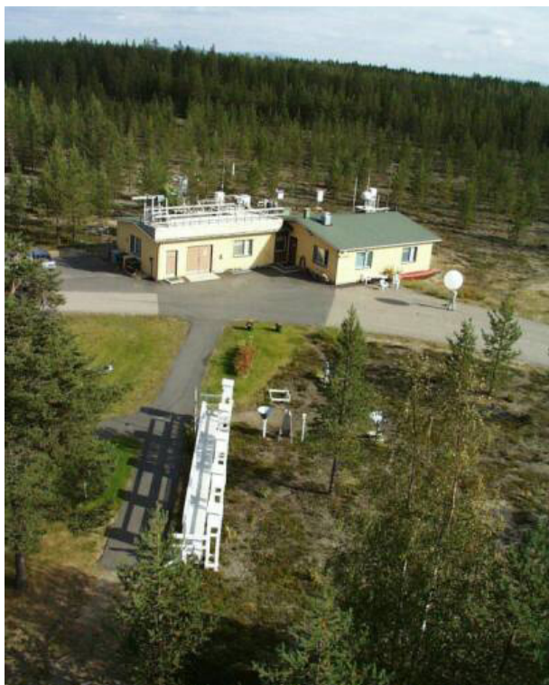
Figure 1. View of Sodankylä observatory. The Brewer is located on the roof in the enclosure on the left.
