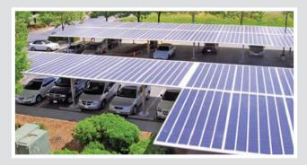
Honeywell Aerospace partnered with Honeywell Building Solutions and the local utility company to install an 840-panel solar canopy, creating 85 covered parking spaces. The system is generating non-grid connected electricity of approximately 350,000 kilowatt-hours of energy annually, which directly feeds the facility. The system displaces nearly 200 metric tons of carbon dioxide, which is equivalent to the annual greenhouse gas emissions generated from 40 passenger vehicles.
