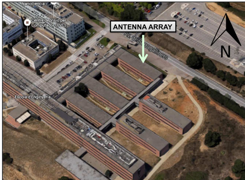
Figure 42 Antenna array location
