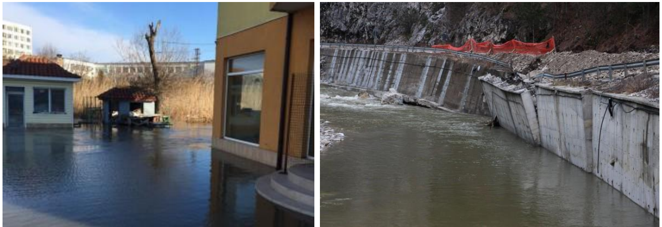
Photo 1 and 2. Photos of floods in Maritsa river basin
