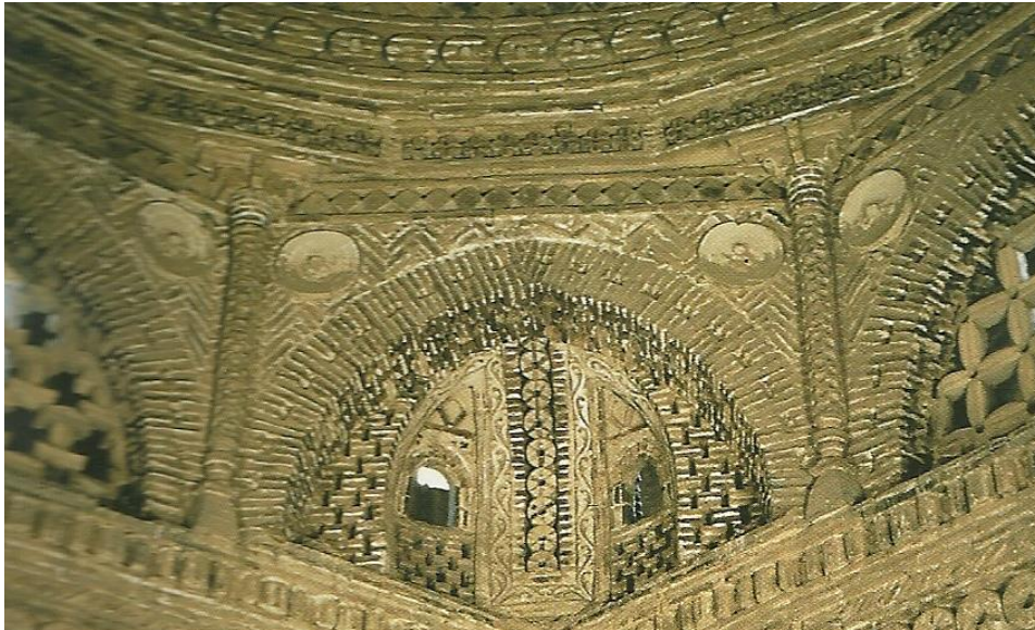
Figure 1: Inside the Sāmānid prince Ismāʿīl Mausoleum at Bukhara –Uzbekistan- (301/914-331/943): the zone of transition. (Photo Christine-Anne Gaillard, in Markus Hattstein et. al., Islam-Kunst und Architektur [Köln, 2000], 115).
