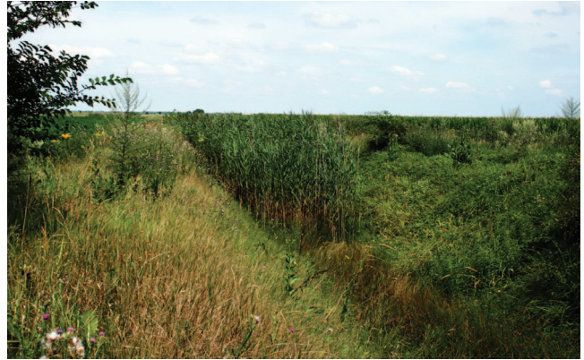
APPENDIX FIGURE 8. Small canal of third order (average width: 1 m) in Sombor municipality, Serbia, that is completely dried out.
