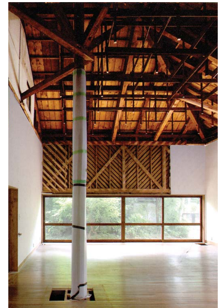
House in White: photo of reconstruction. The hidden and the visible.
