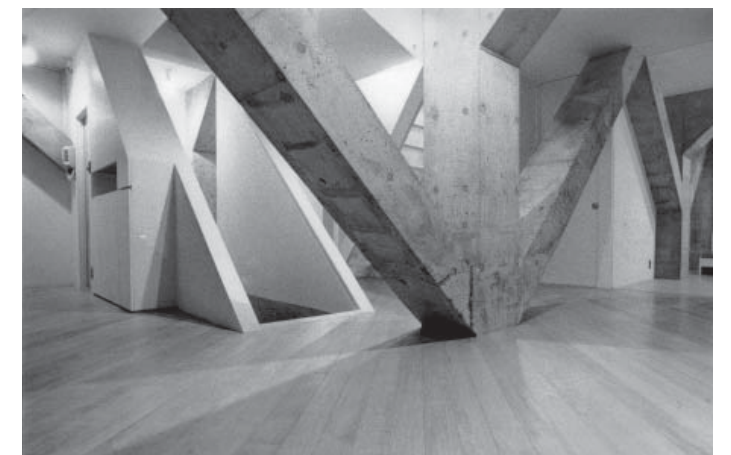
House in Uehara: construction of the shell, and finished result
