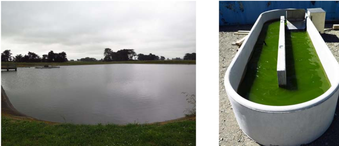
Image 1.3 Microalgal open systems. Left: facultative pond; Right: High Rate Algal Pond.
