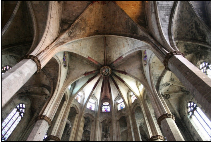
Figure 4.4 Ribbed vault between the apse and the presbytery
