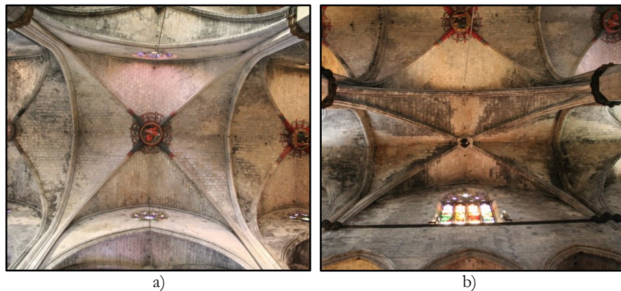
Figure 4.3 a) Crossed vaults in central nave; b) lateral nave
