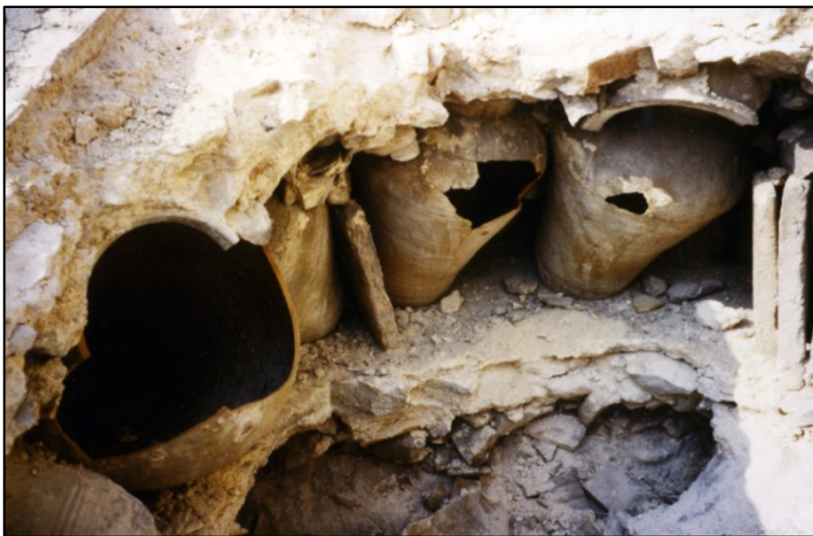
Figure 4.6 Pottery filling over the central vaults
