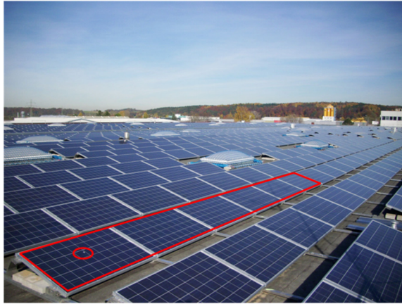
Fig 1.3 Example of a PV plant, the red lines indicate respectively a single PV cell and one PV string.
