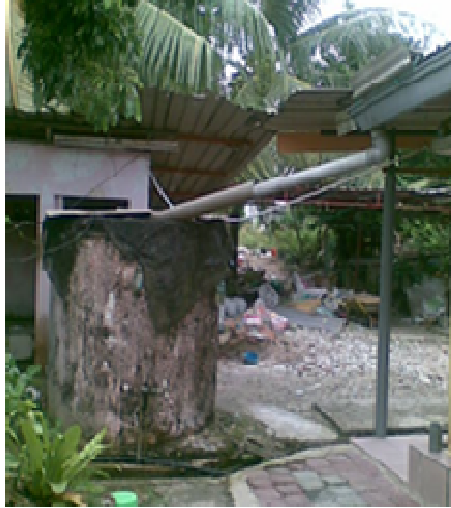
Figure 1.7 Rainwater harvesting for non-potable usage (Rosli, 2010)
