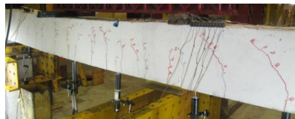
Fig. 7. Experimental crack distribution at load 133 kN
