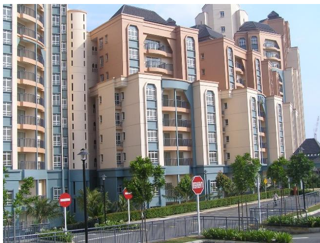
Figure 1 Precast concrete buildings constructed using precast concrete wall components
