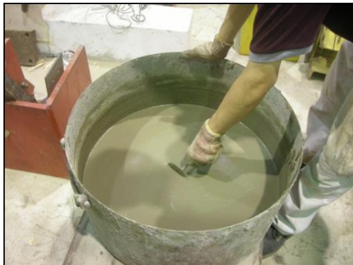
Figure 4 Preparation of grout
