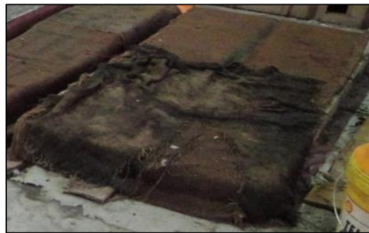
Figure 2 Burlaps used for the wet curing
