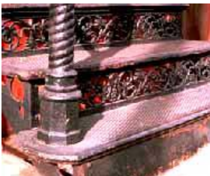
Figure 4 Cast iron steps with highly decorative patterns
