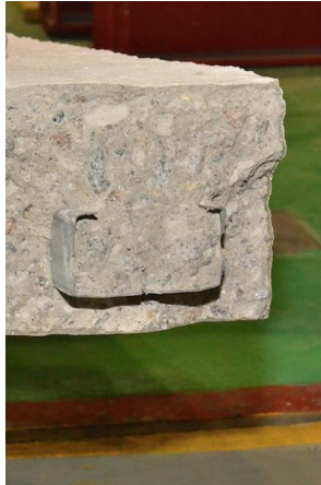
Figure 5 Tearing of shear connector
