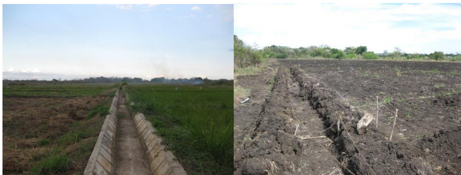
Figure 9. Left: Concrete irrigation canal in the rice scheme in Misasi. Right: Soil irrigation channel in the rice scheme in Kakora. (Photo: Agnar Kjeller).
