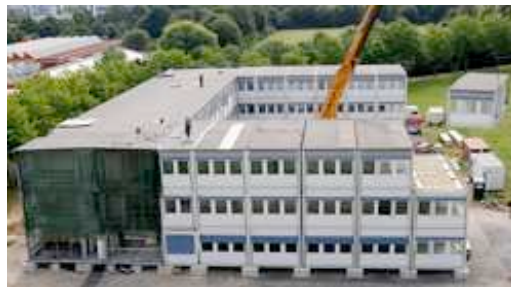
Figure 1: A part of Bielefeld University is built from container modules.
