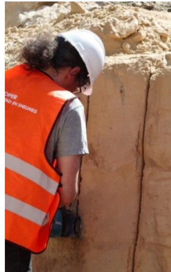
Figure 5.22. Mechanical cutting of the rock
