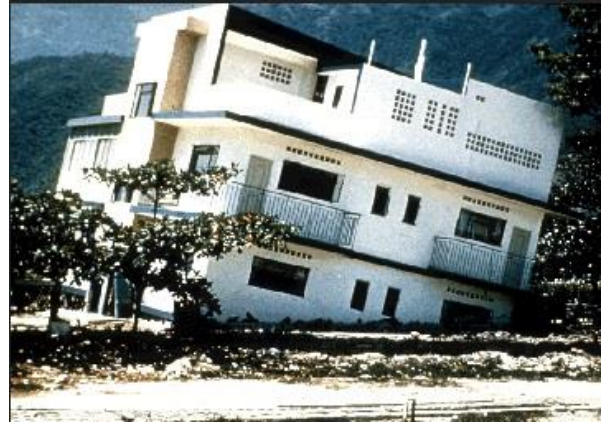
Figure 2.6. Liquefaction induced by earthquake (Venezuela 1967)
