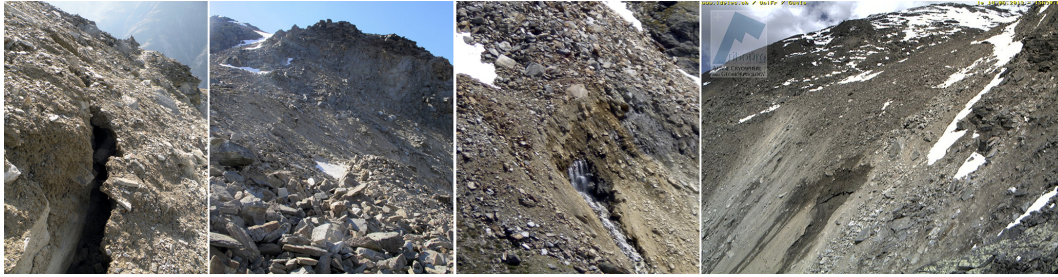
Figure 10. Visible cracks (left, from September 2011) and depressions (middle left, from June 2013) at the front of the rock glacier Breithorn, visible water outflow (middle right) at the front of rock glacier Dirru (from June 2013), and a webcam image of the front of rock glacier Breithorn (right, from 14 June 2013).
