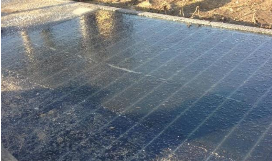
Figure 5-9: High reflectance of the solar road (Hruska, 2014)
