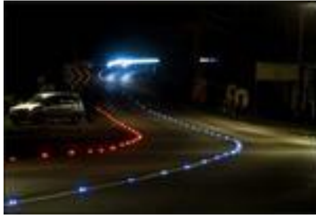
Figure 5-14: Solar cat-eyes (Lighting Matters, 2015)
