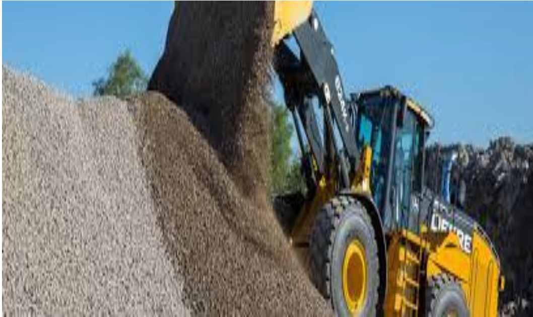
Figure 5-31: Re-Sand Bauxite Residue in Road Construction (Evans 2011)
