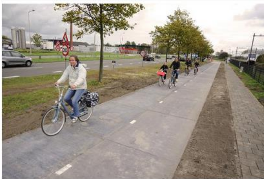
Figure 5-7: Test usage of the Bike Solar Road (Hruska, 2014)
