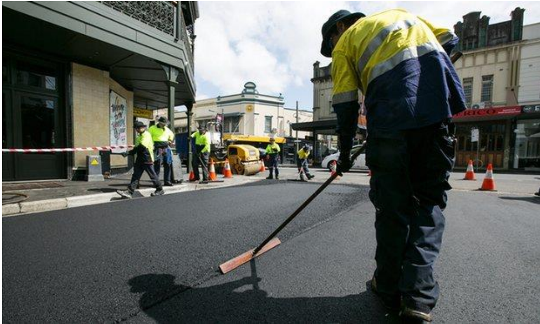
Figure 5-25: Re-surfacing using asphalt containing recycled printer toner (City of Sydney, 2015)
