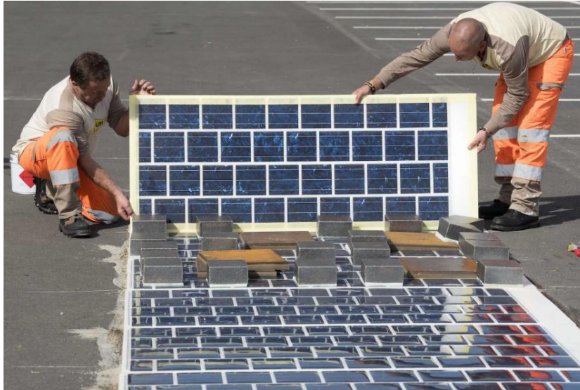
Figure 5-10: Installation of solar panels in France (Wang, 2016)
