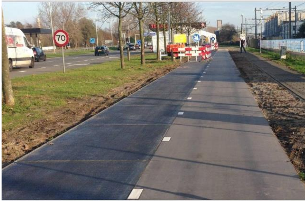
Figure 5-8: The Bike Solar Road (Hruska, 2014)
