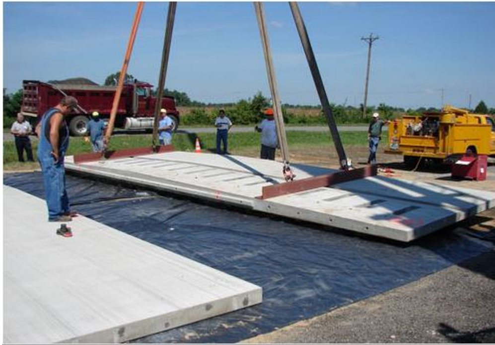
Figure 5-23: The PPCP over polythene sheet (D. K. Merritt & Tayabji, 2009)
