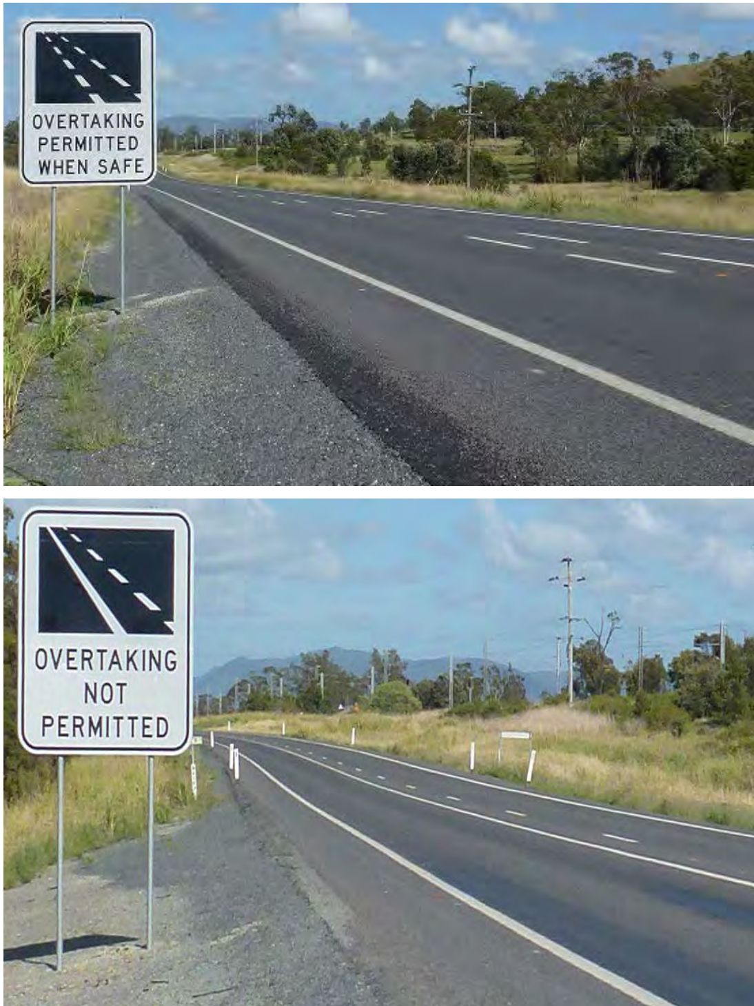
Figure 2.4 Photos of WCL treatments - Miram Vale to Rockhampton
