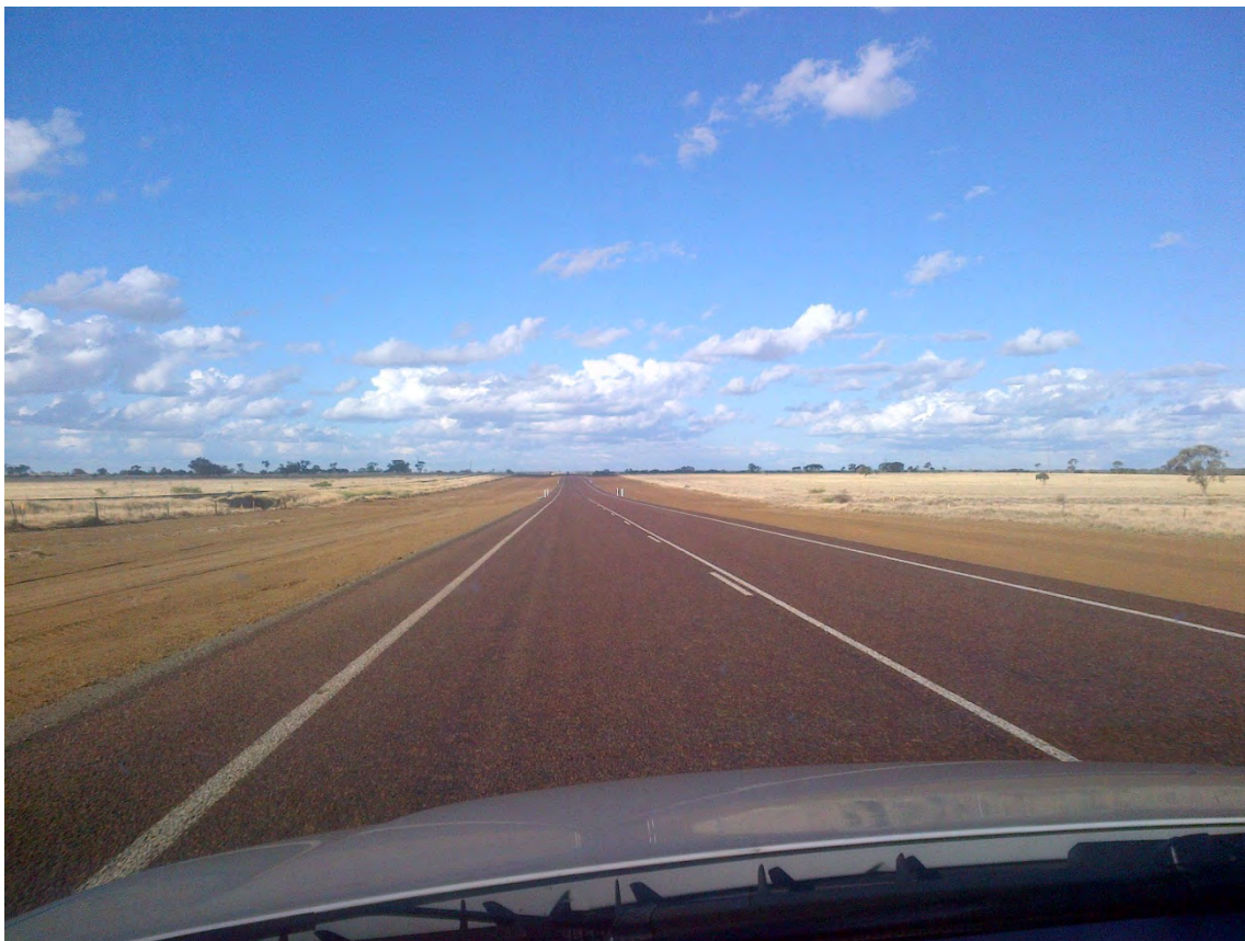
Figure 2.3 Photo of a Clear Zone Project in Western Queensland
