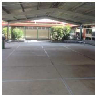
Figure 4.4. Undercover area, facing towards toilet block (Mem)
