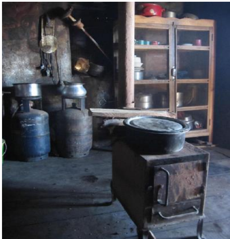
Figure 6.4: A bukhari used for space heating, made of metal and with a chimney. It can also be seen an evident fuel stacking taking place in this house.
