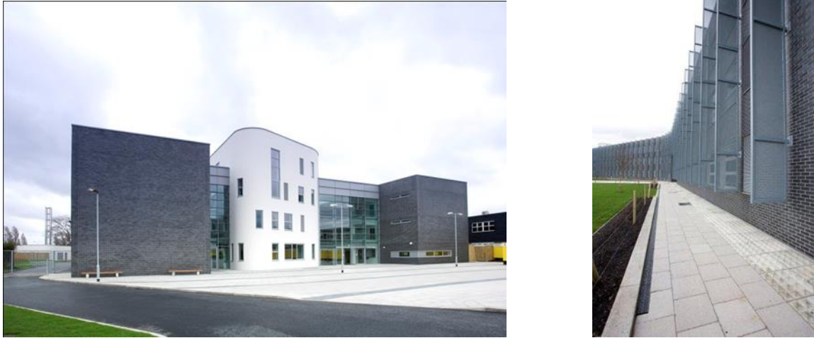
FIGURE 2. Building A entrance (left, north facade), and vertical shading (right, west facade)
