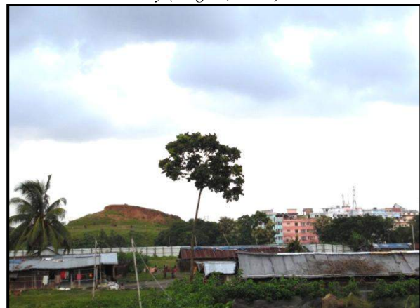
Figure 2.22: Tin shed housing and Multistoried buildings around Red hill Source: Field Survey (August, 2014)
