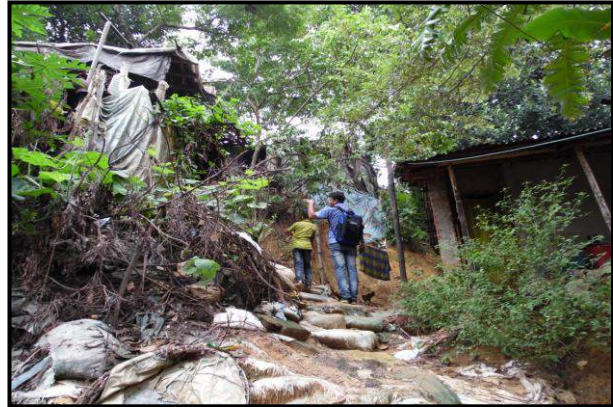
Figure 2.29: Houses are constructed through hill cutting in Goachi Bagan Hill, pachlish Source: Field Survey (August, 2014)
