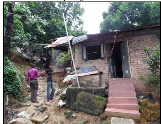
Figure 2.48: Housing at Goachi Bagan area. Source: Field Survey, August, 2014
