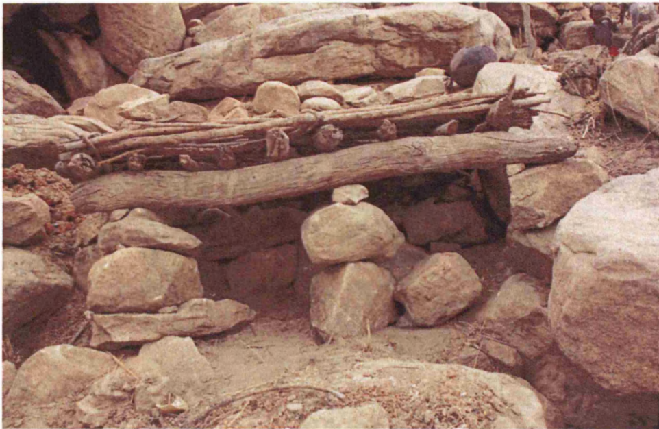
Fig. 8.8. Foundation cross-section
