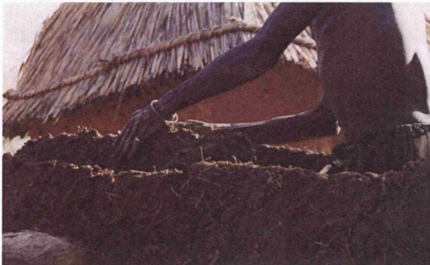
Fig.8.26 Flattening the walls
