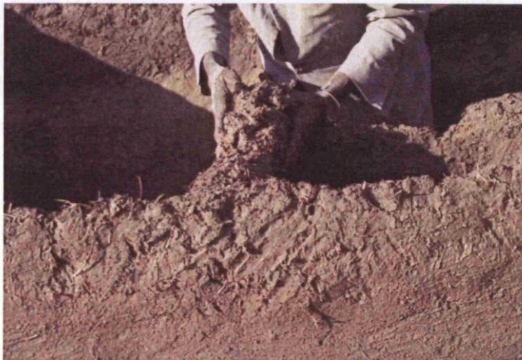
Fig.8.24 Stabilizing the walls
