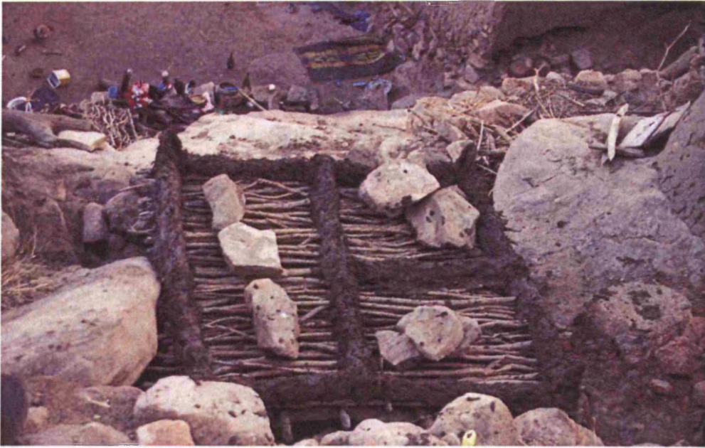
Fig.8.14 Overview of the construction site with four ama corners
