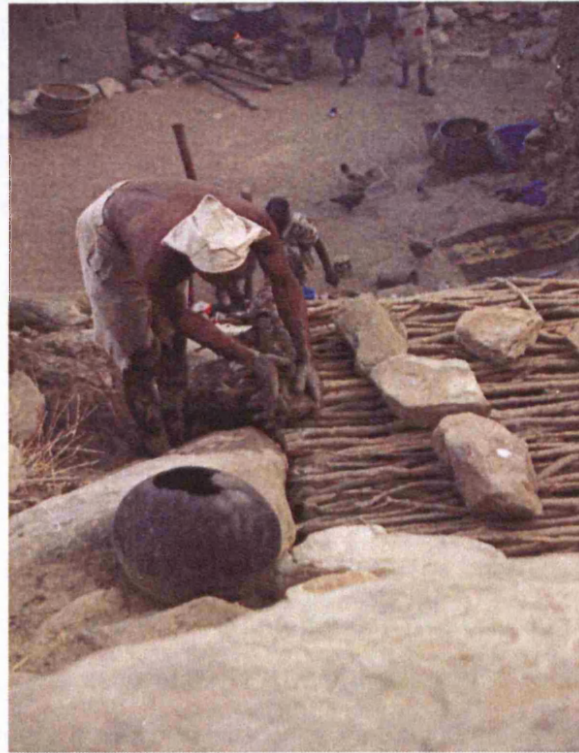
Fig. 8.9. Starting to build the wall
