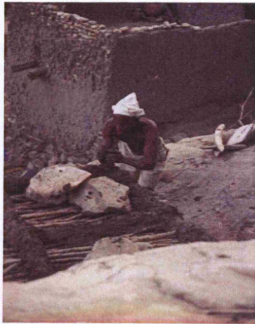
Fig.8.13 Fixing the ama corner
