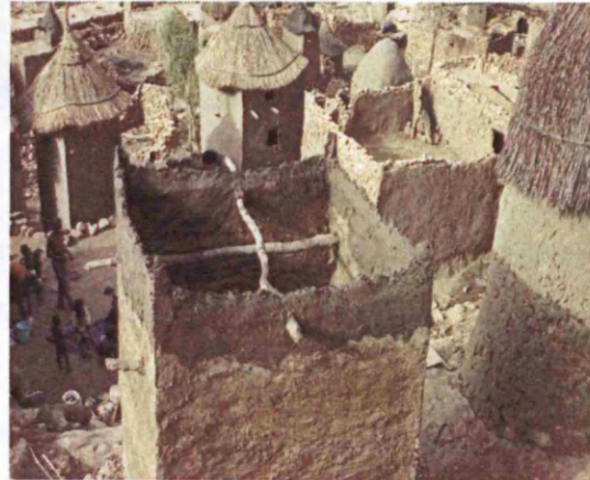
Fig.8.35 Base of the upper compartments
