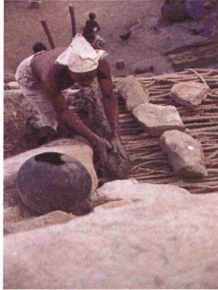
Fig.8.11. Attaching the mud
