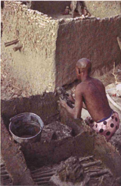
Fig. 8.15. Fixing the mud on the cone
