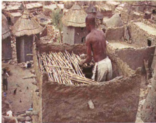
Fig.8.36 Laying out millet straws
