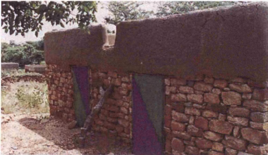
Fig.6.7. Gujo with painted doors
