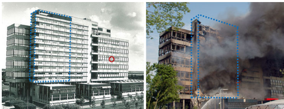
Figure 4. Fire origin (red circle) and collapsed portion of the building (blue dotted lines) [19, 20] (Color figure online).
