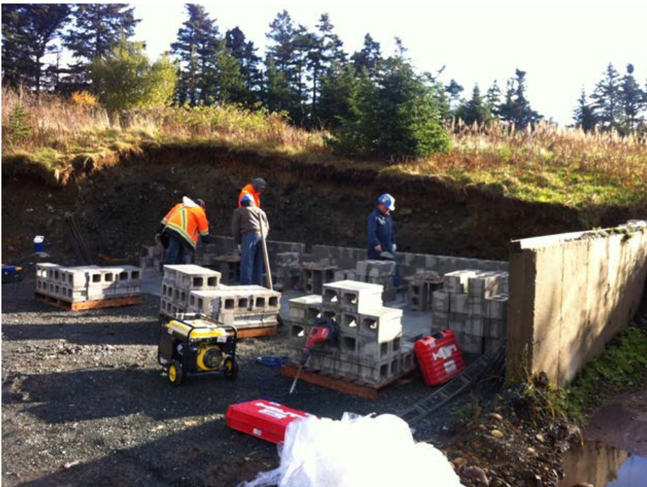
#2 - Compost platform wall construction
