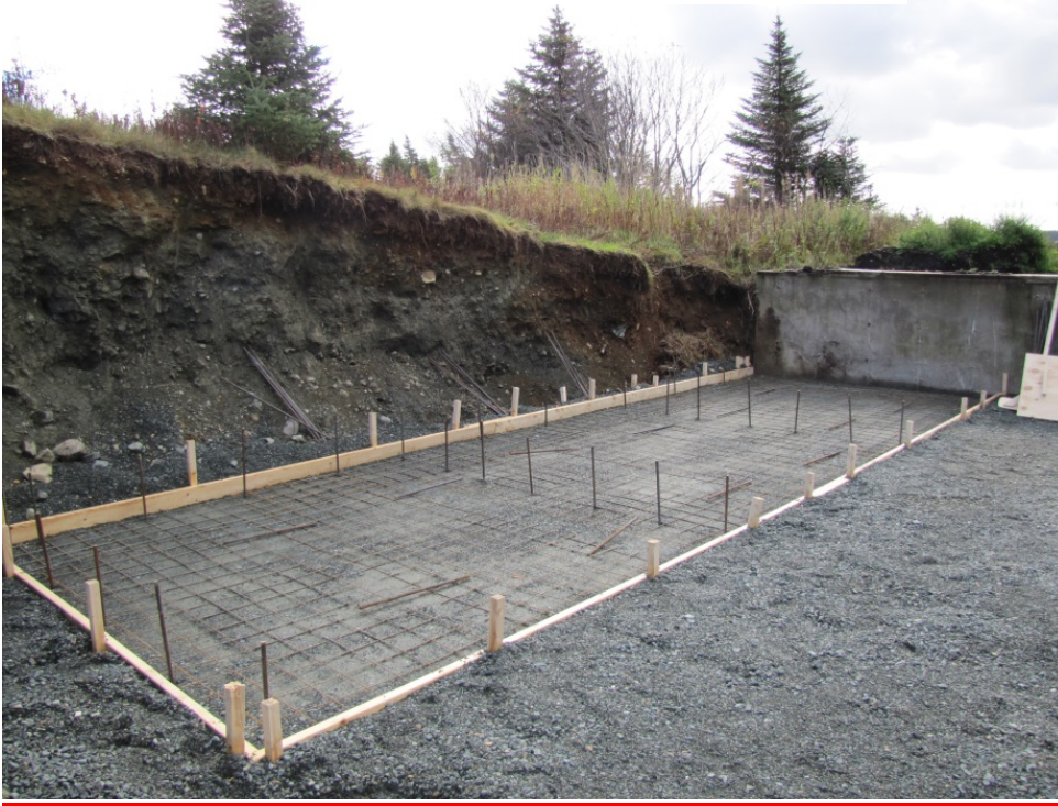
#1 – Compost platform floor construction
