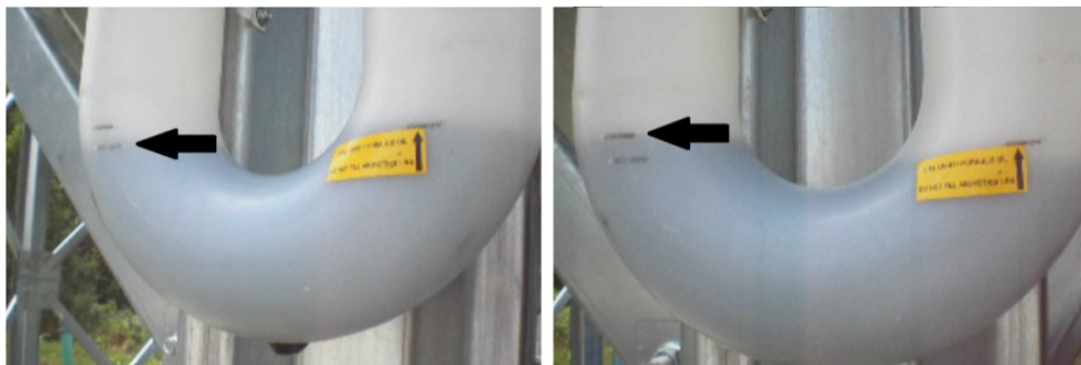
Figure 3.5 U-shape pressure relief valve used as a monitor during a pressure decay test showing the silo before pressure was induced (left) and pressurized to approximately 170 Pa (right).
