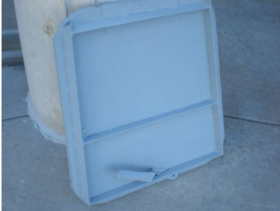
Figure 3.13 Reinforced entry hatch door installed on one of the roof panels.
