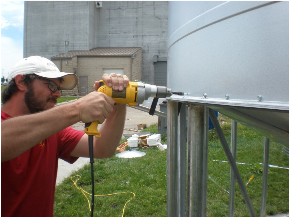
Figure 3.30 The author attaching the Bird's silo to its base assembly using self-tapping screws.
