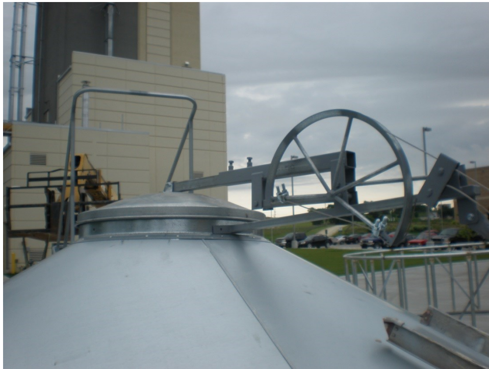
Figure 3.23 The roof cap opening and closing apparatus designed to provide an airtight seal with the help of a winch operated from ground level.
