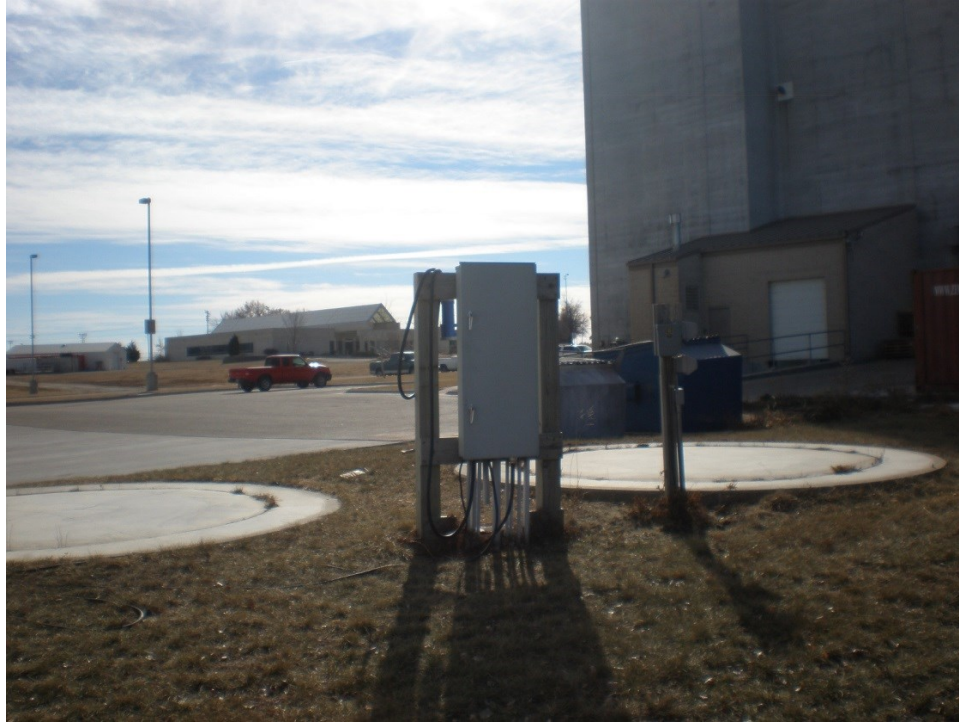
Figure 3.2 Site of silo construction and placement at Kansas State University, Manhattan, KS.
