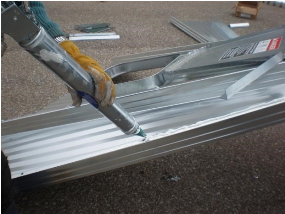
Figure 3.7 Placing sealant along the overlapping ribs between roof sections.
