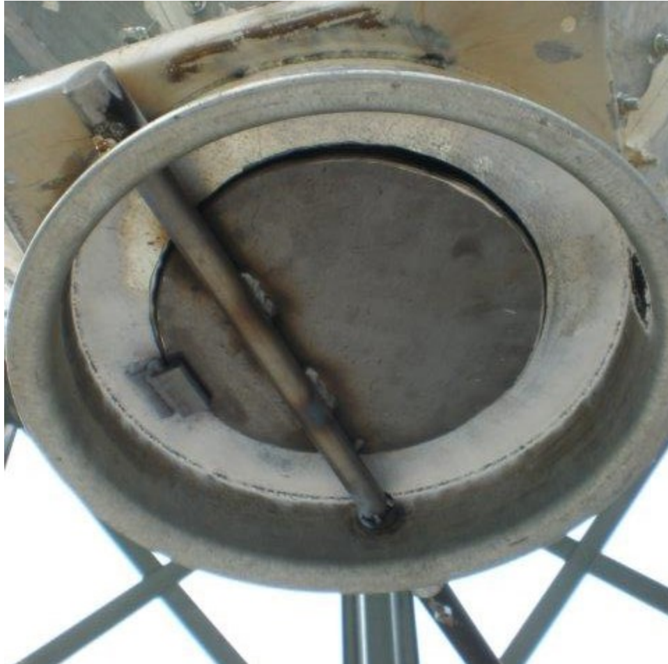
Figure 3.31 Butterfly valve installed at the bottom of the silo hopper cone for discharging the grain. The narrow gap around the opening allows fumigant in and out of the \text{PH}_3 reaction chamber installed below (see Figure 32).
