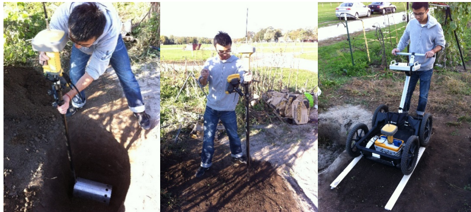
Figure 4.26 Buried depth measurement using RTK GPS and GPR
