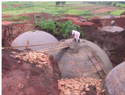
Figure A.30: Exterior plastering
