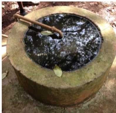
Figure A.41: Properly applied water bath
