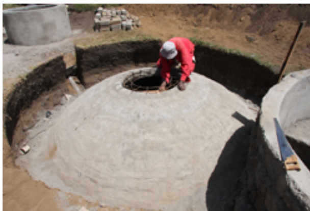
Figure A.27: Upper dome top opening
