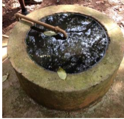
Figure 3.4: Properly sealed digester lid
