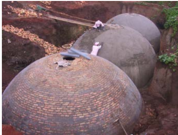
Figure A.3: Digesters in series
