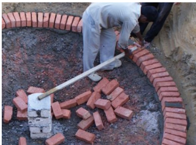
Figure A.6: Using the guide stick Mixing mortar/plaster and concrete
