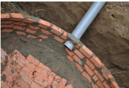
Figure A.14: Pipe positioning
