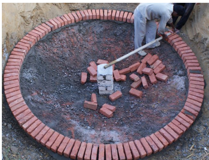
Figure A.11: Reinforcement ring
