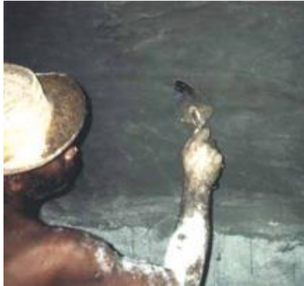
Figure A.17: Interior plastering
