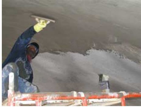
Figure A.29: Interior plastering
