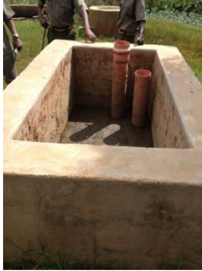
Figure A.40: Inlet Mixing Chamber
