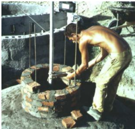
Figure A.36: Neck construction process
