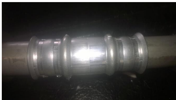
Figure 1: Aluminum flame-free fitting installed on a 15.9 mm tube
