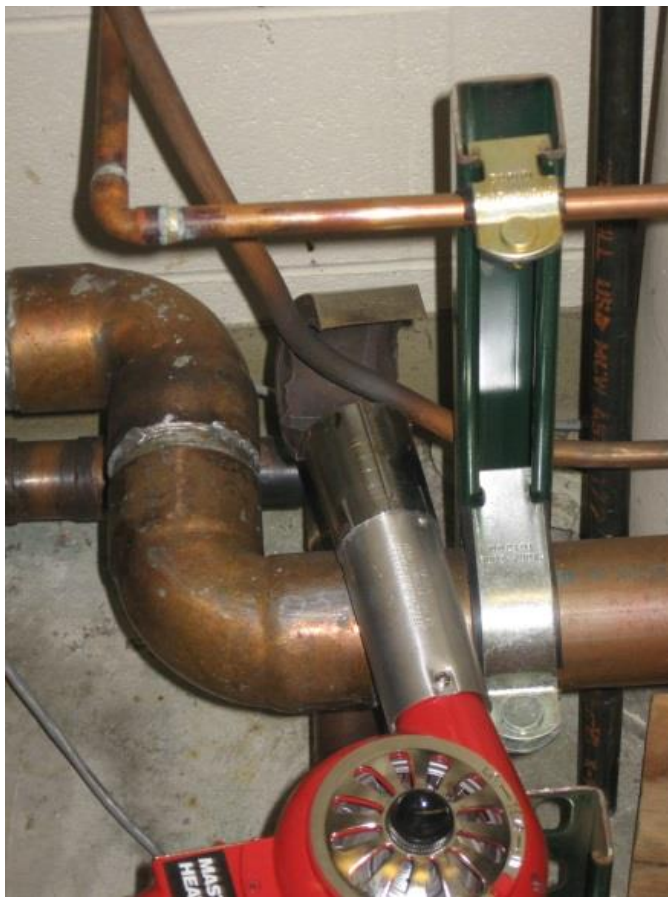
Figure E.6. Heat gun used to keep the gas meter from freezing.
