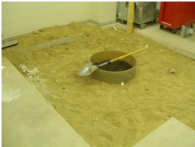
Figure 3.3. Lab space during construction of the pit.
