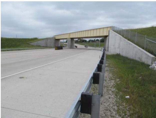
Figure 3.2 Bridge overpass on 231Route.
