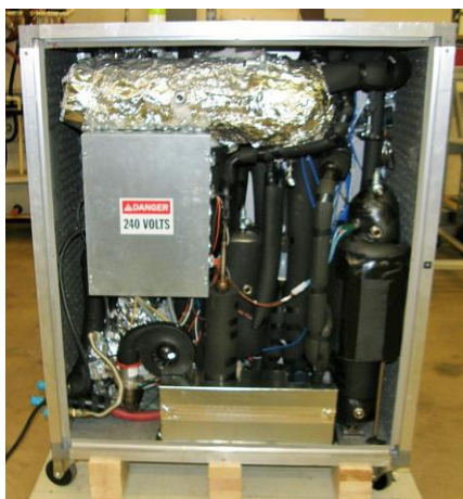
Figure 2: Heat pump components housed within unit
