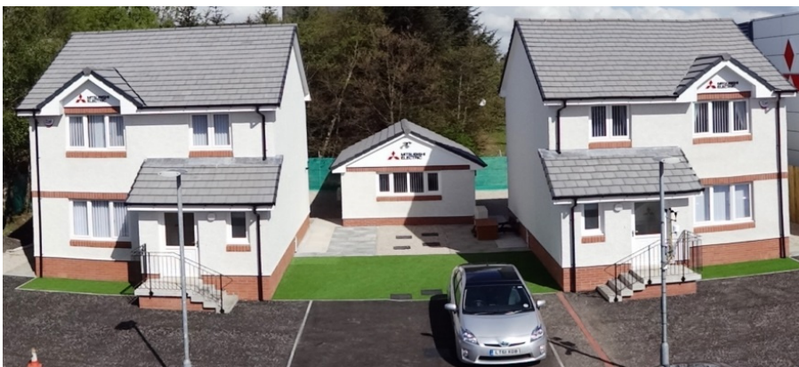
Figure 2: Mitsubishi Electric House-type Evaluation Facility
