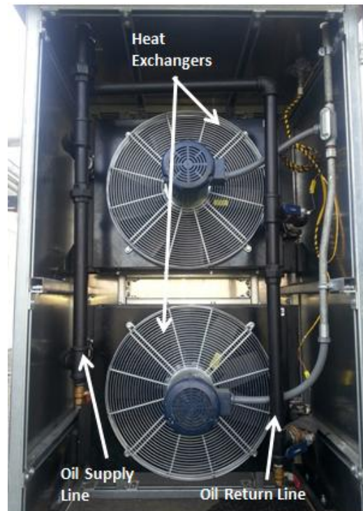
Figure 2.12: Outdoor heat exchanger layout.
