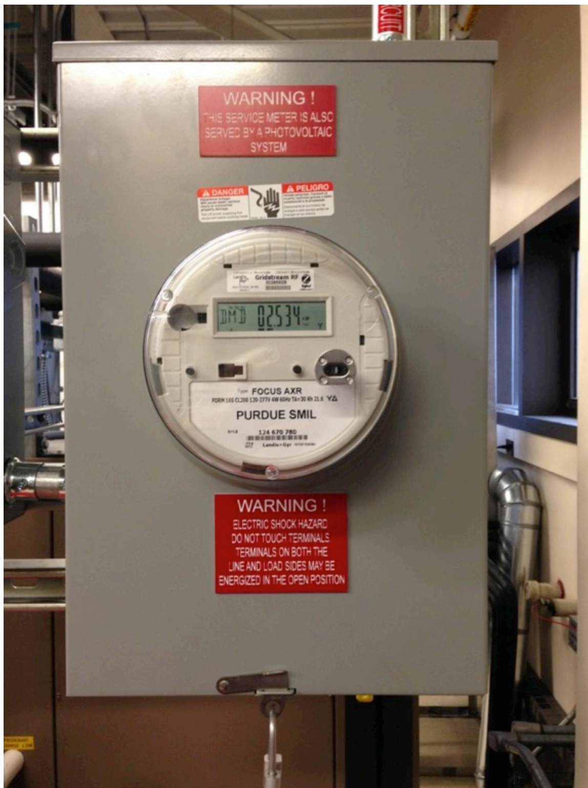
Figure C.9 Landis+Gyr E330 FOCUS AX Polyphase Smart Meter
