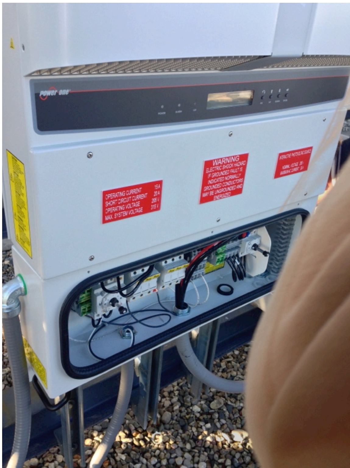
Figure C.14 Wiring Installation for Power-One Inverter
