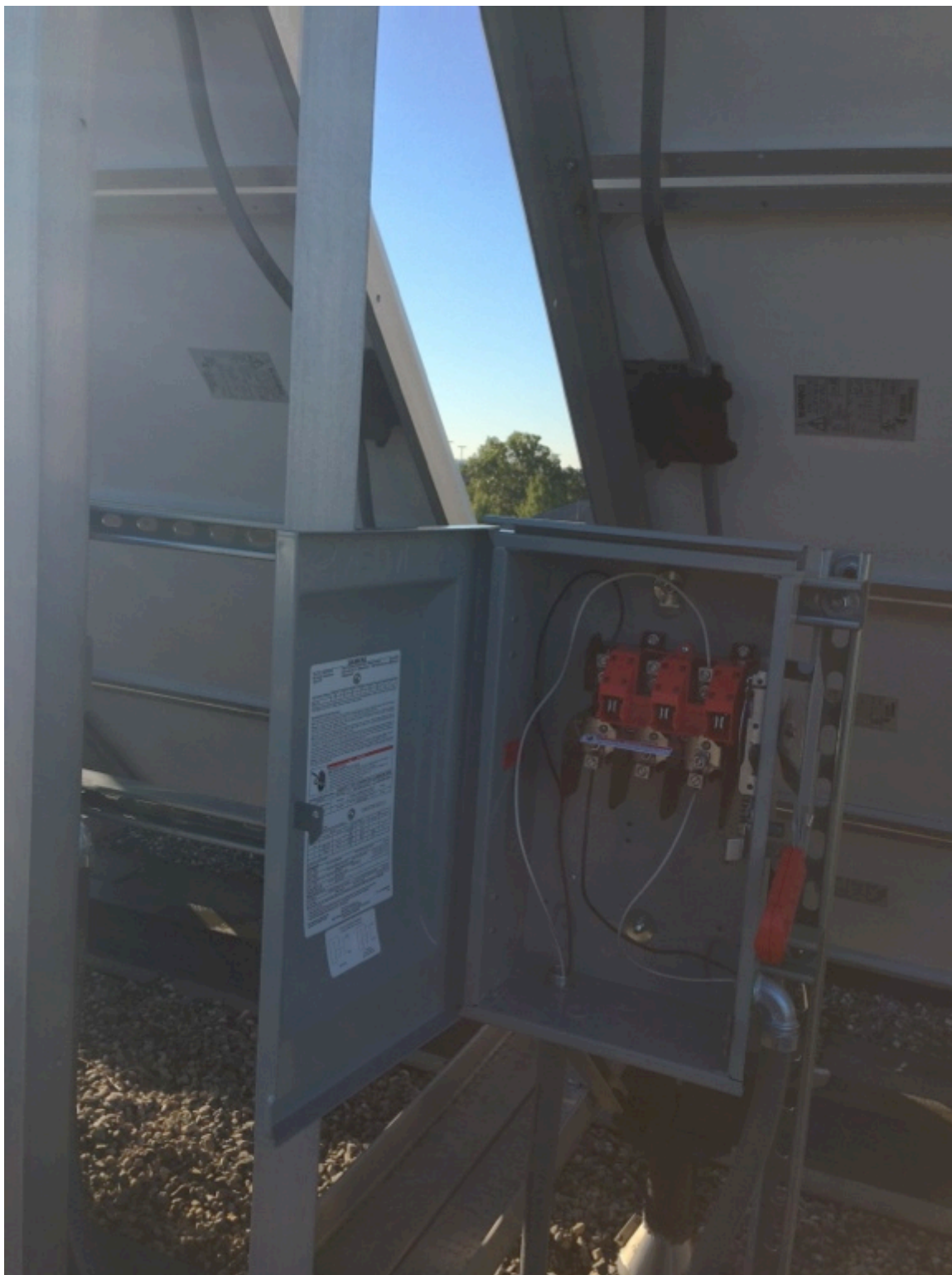
Figure C.15 Wiring Installation into DC Disconnects from Sub-Arrays
