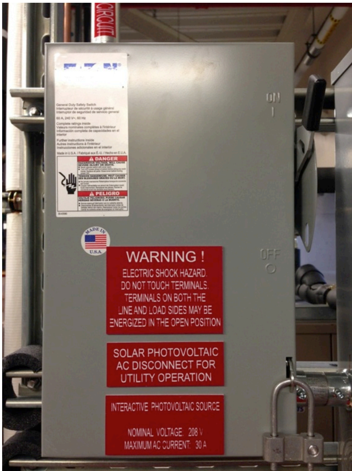
Figure C.10 Eaton 250VAC 60A Fused AC Disconnect
