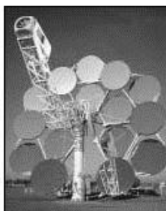
This dish/Stirling solar power system in Arizona is capable of producing 25 kW of electricity.
