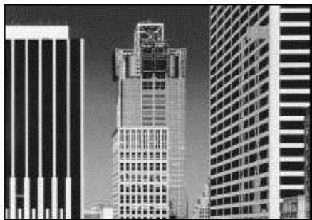
The Four Times Square Building in New York City uses thin-film PV panels to reduce the building's power load from the utility grid.
