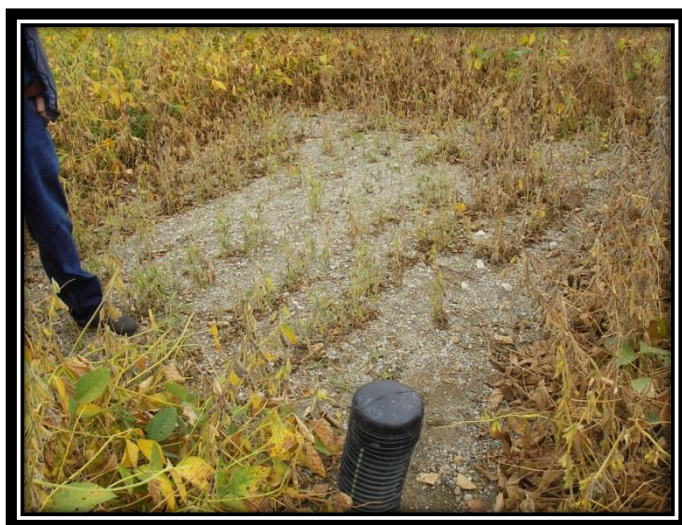
Figure 1. Blind inlet and a tile riser on a field with a soybean crop.
