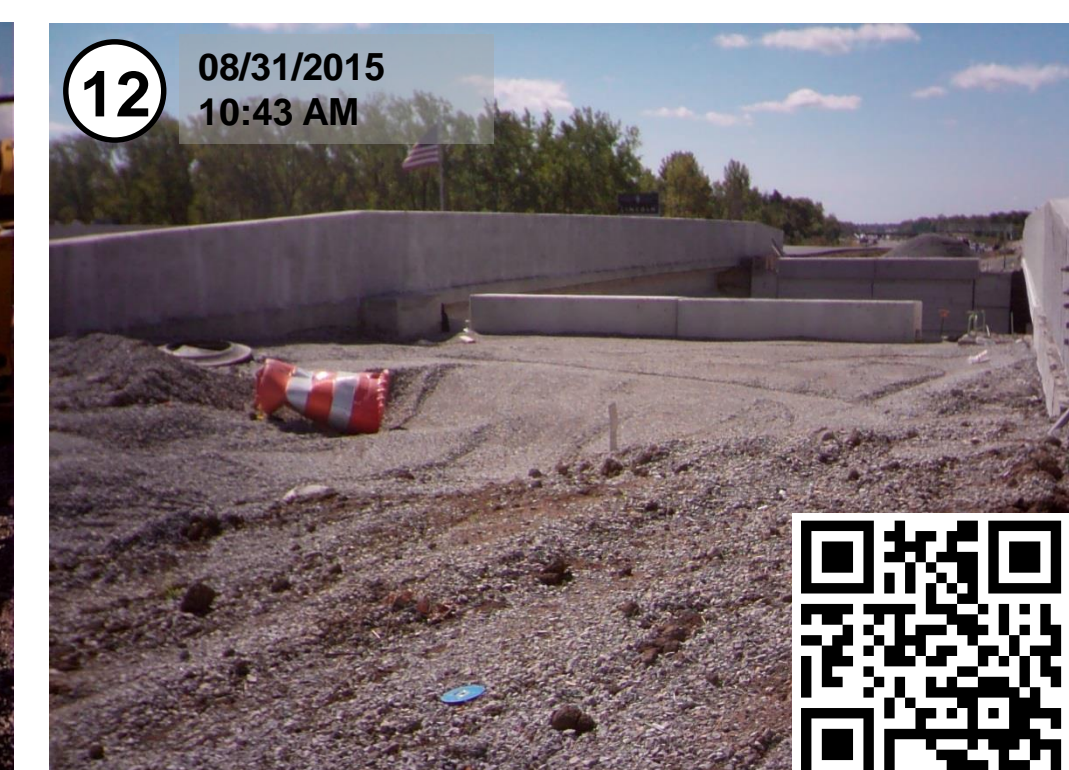
Concrete cures - Bridge is complete
