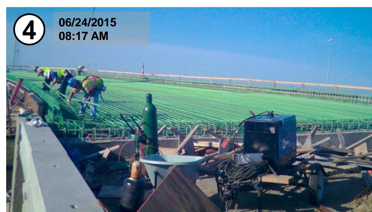
Bridge deck steel reinforcement being placed
