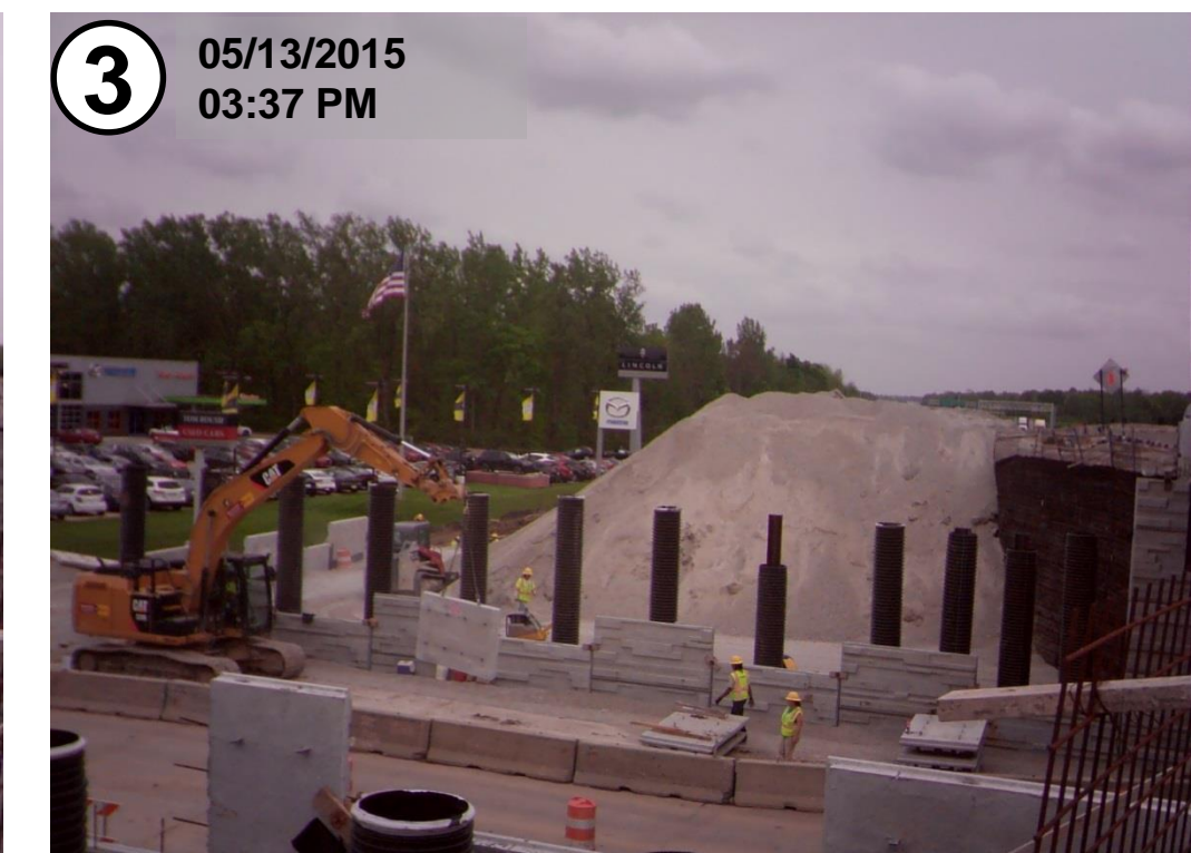
MSE Wall construction - panel placement
