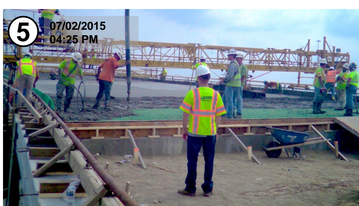
Concrete is placed on the bridge deck
