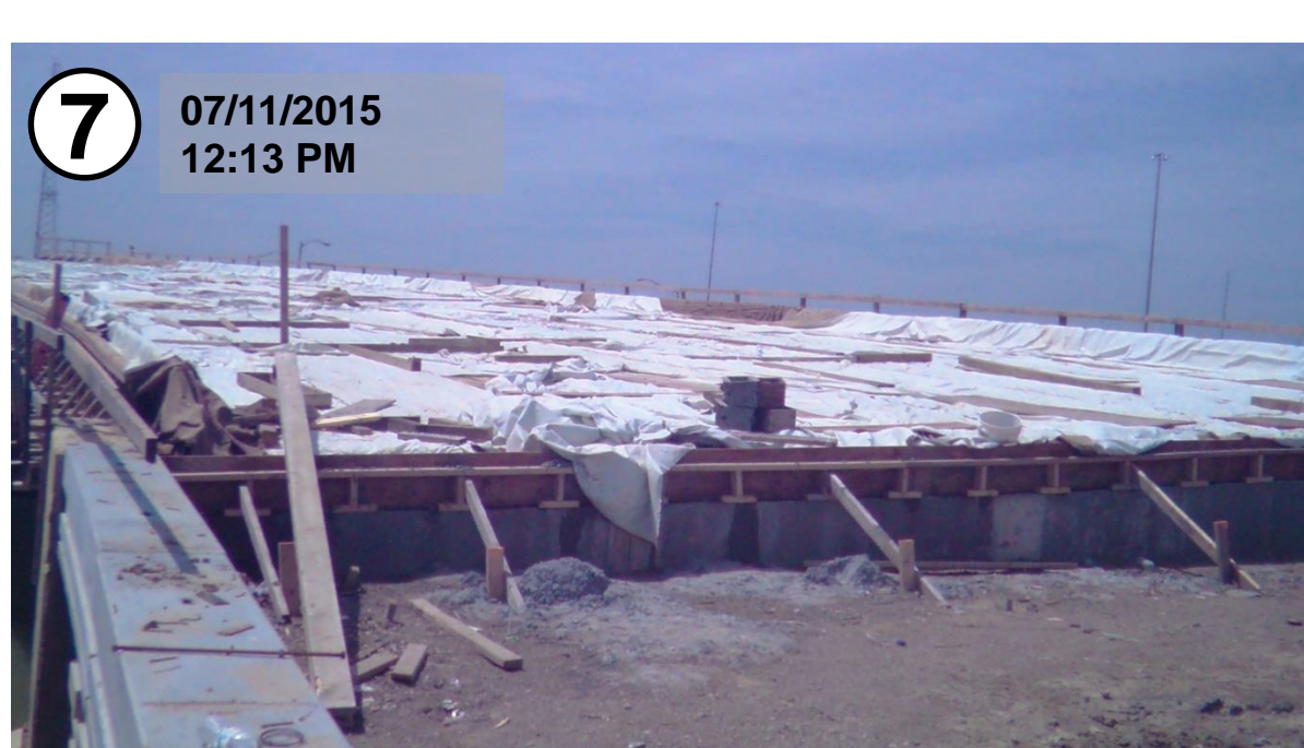
Concrete cures in accordance with INDOT standards
