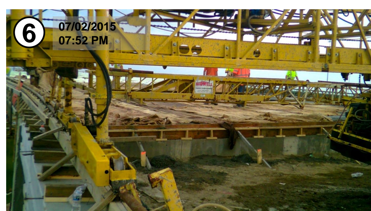
Concrete is covered with burlap for curing process
