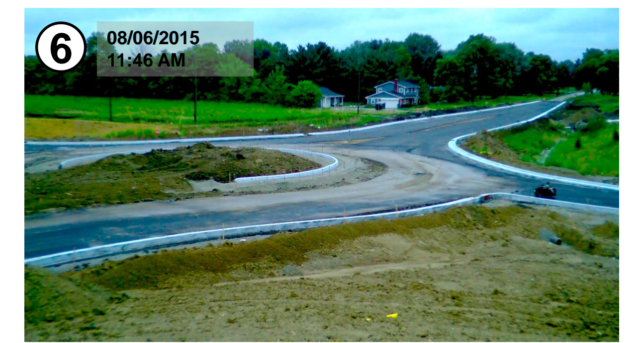
Concrete shoulders are slip-formed
