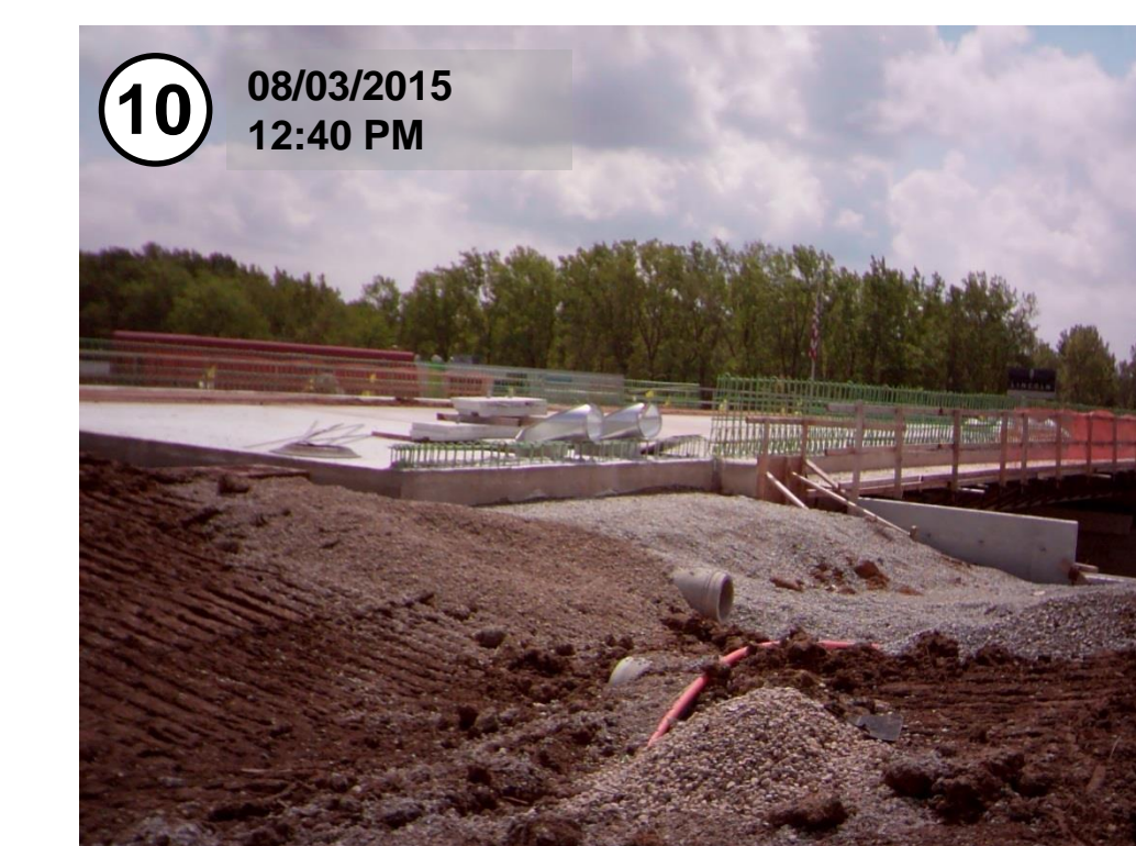
Steel is laid out for concrete safety barrier
