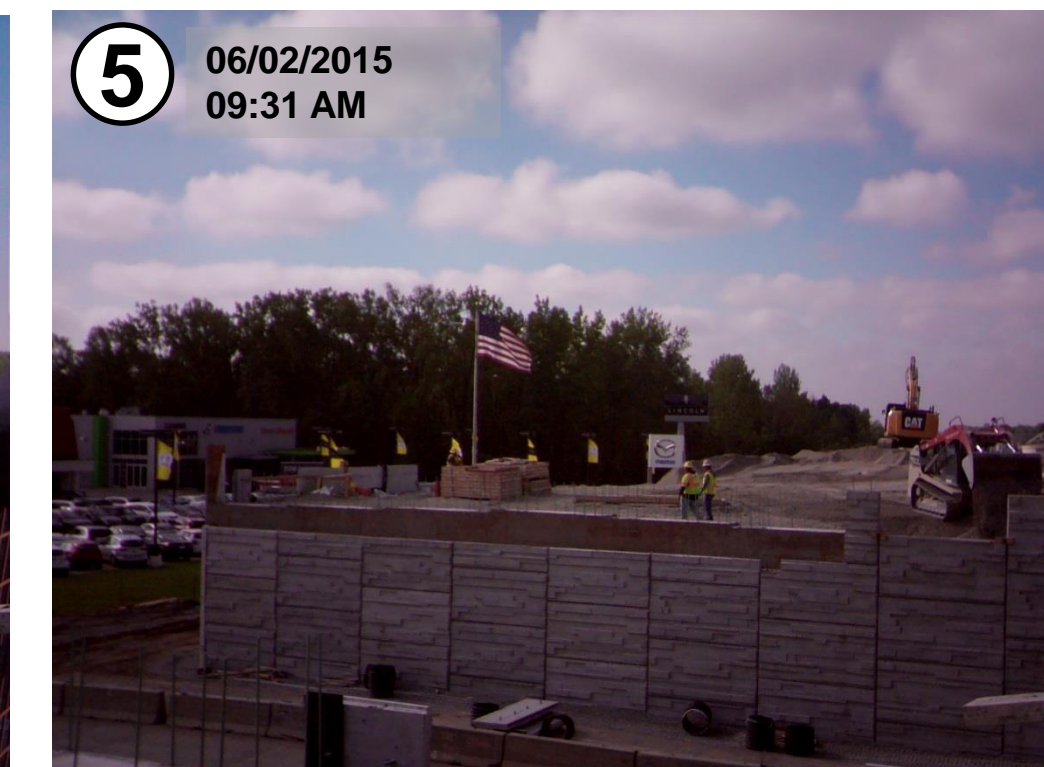
MSE Wall complete - Beam seats constructed
