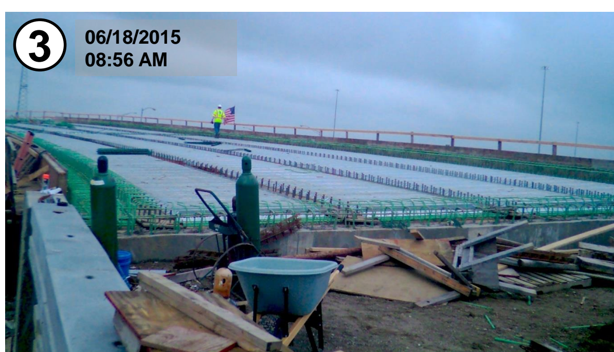
Beginning of steel layout on bridge deck
