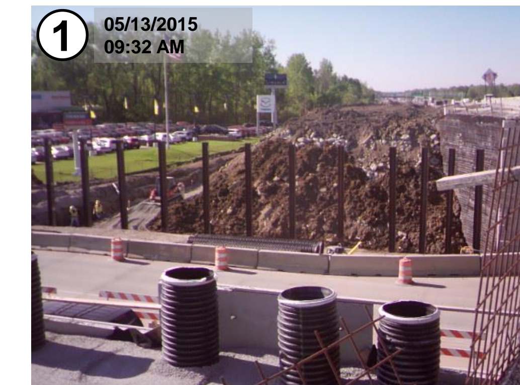
H-Piles are driven; preparation for MSE Wall
