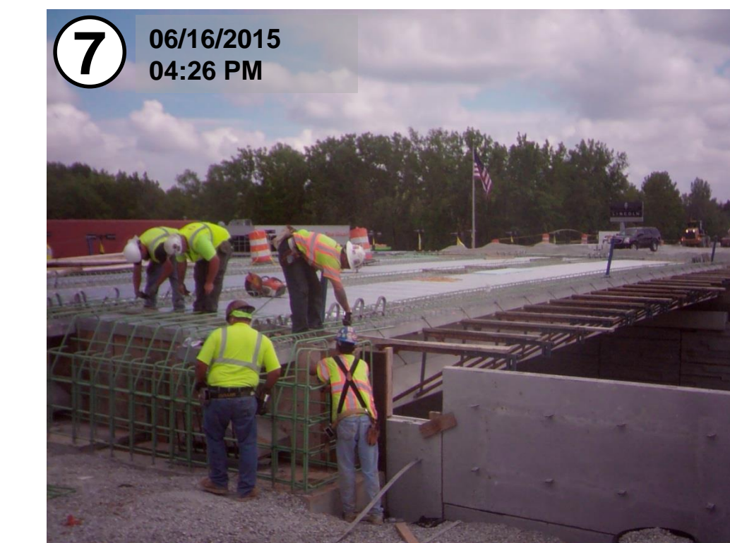
Bridge deck construction
