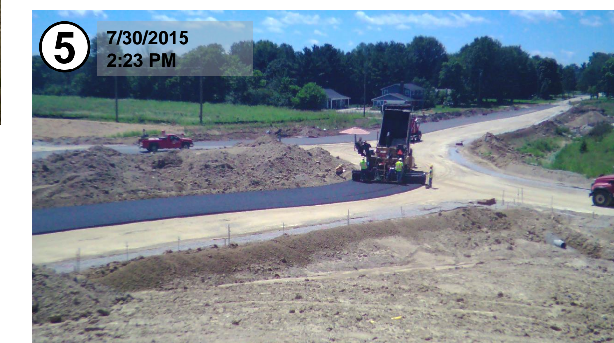
Hot Mix Asphalt base layer is constructed
