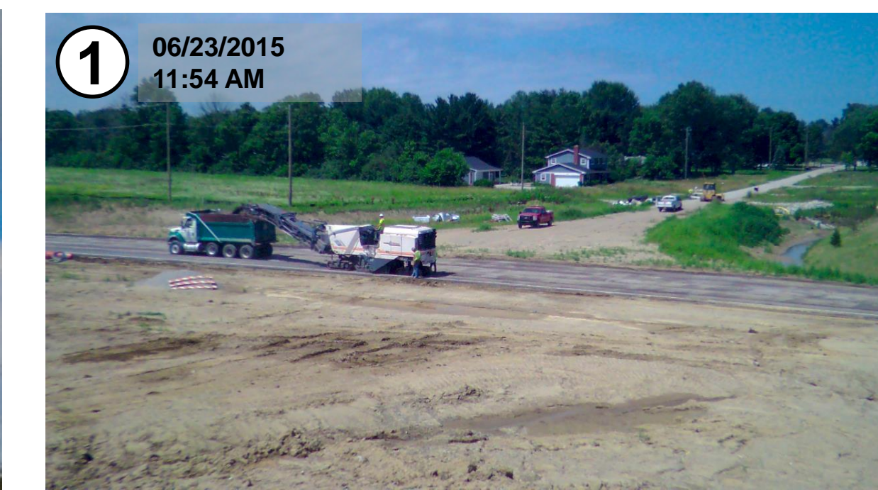
Existing road is removed by asphalt milling machine
