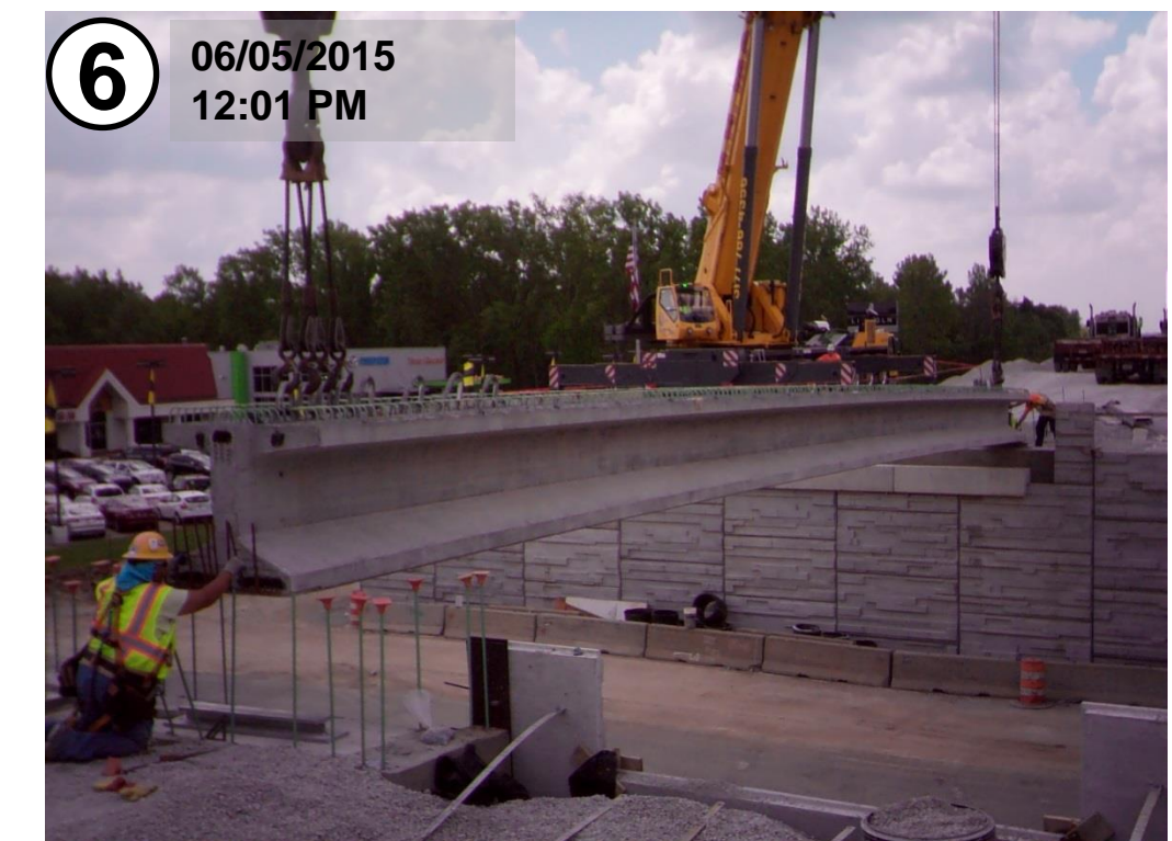
Concrete bridge beam placement
