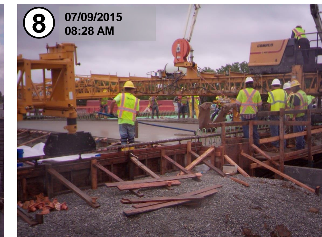
Concrete is poured for bridge deck
