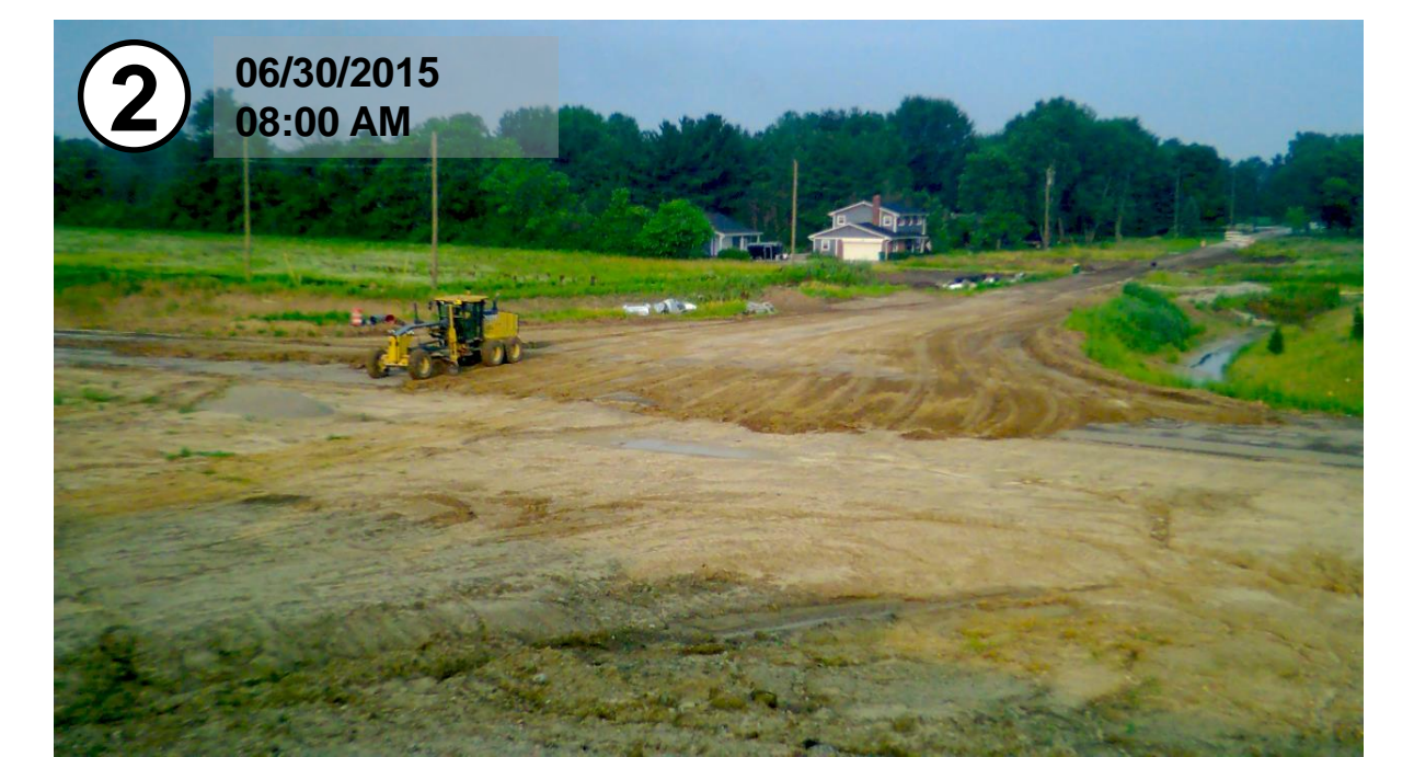
Earthwork begins on the construction site
