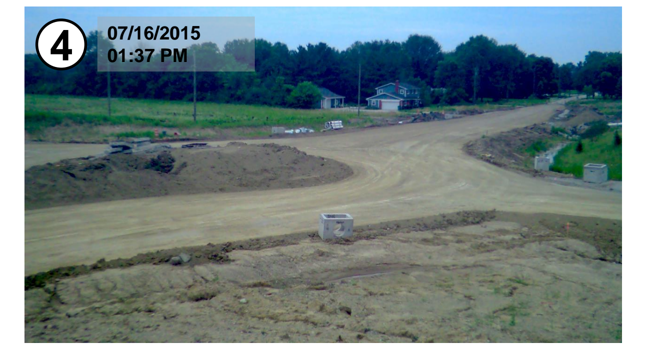
Soil stabilization process is completed
