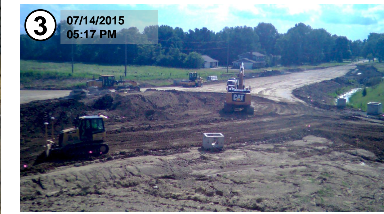
Earthwork and grading continue
