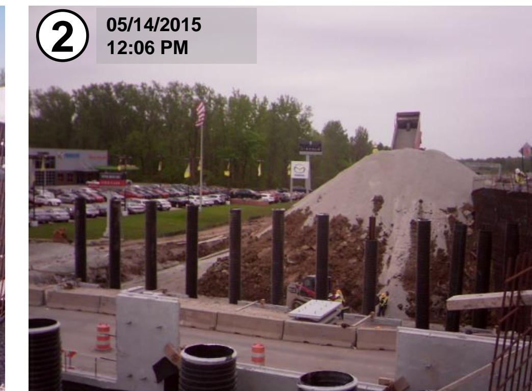
Structure backfill placed for MSE Wall
