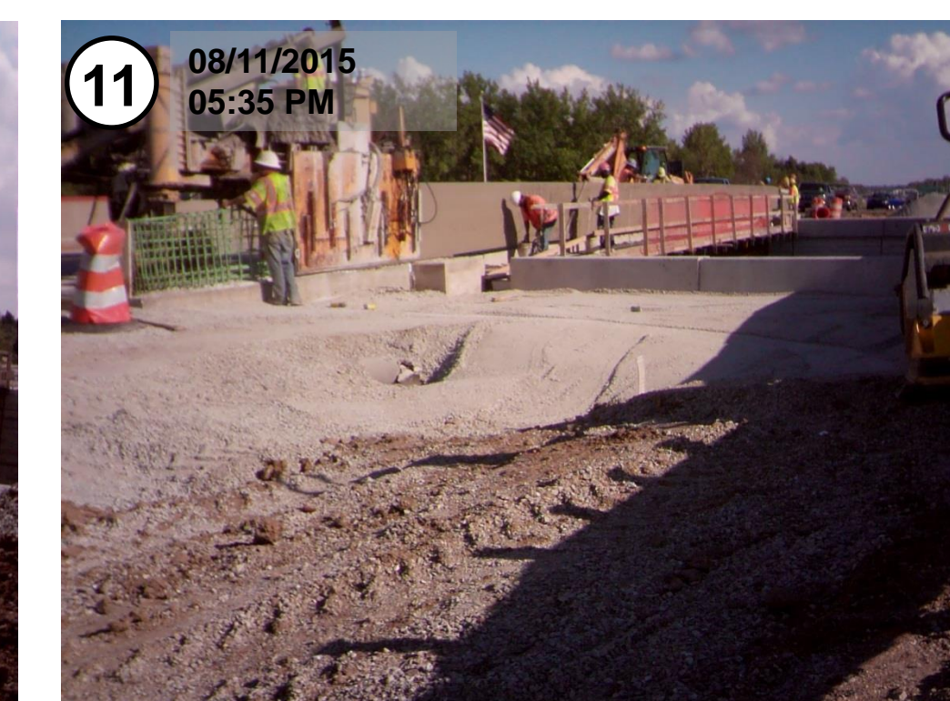
Concrete safety barrier is slip-formed
