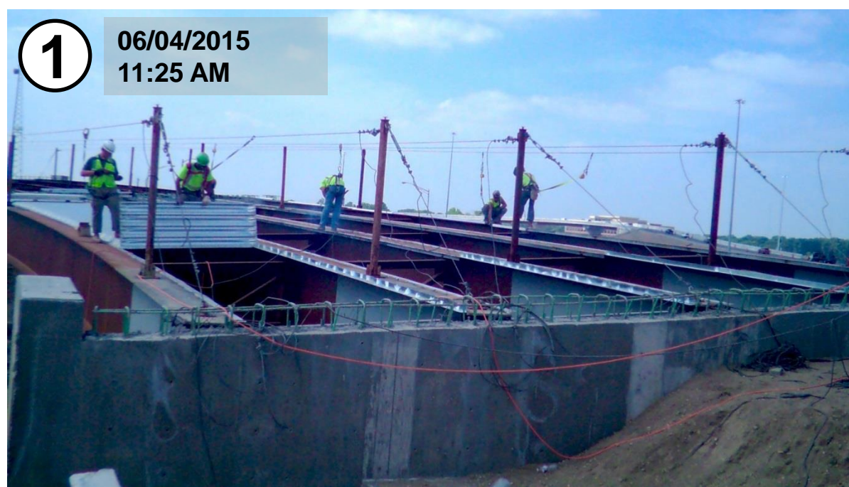
Deck pans being placed on steel bridge beams
