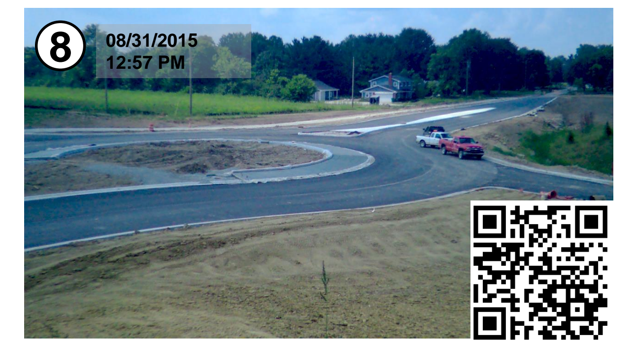
Construction continues on site
