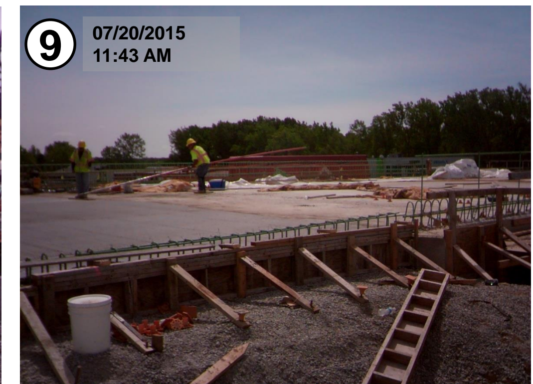
Concrete is poured for bridge approach slab
