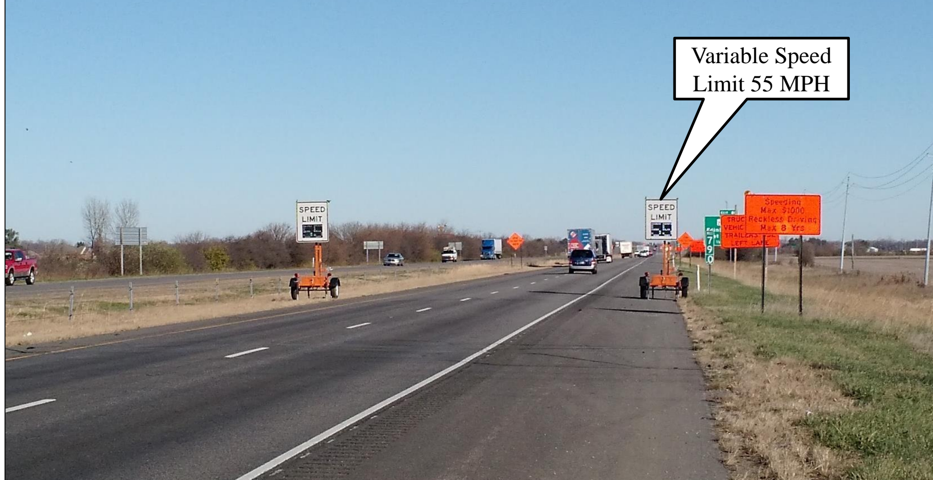
Paired Variable Speed Limit Signs at I-65 NB Mile Marker 79
