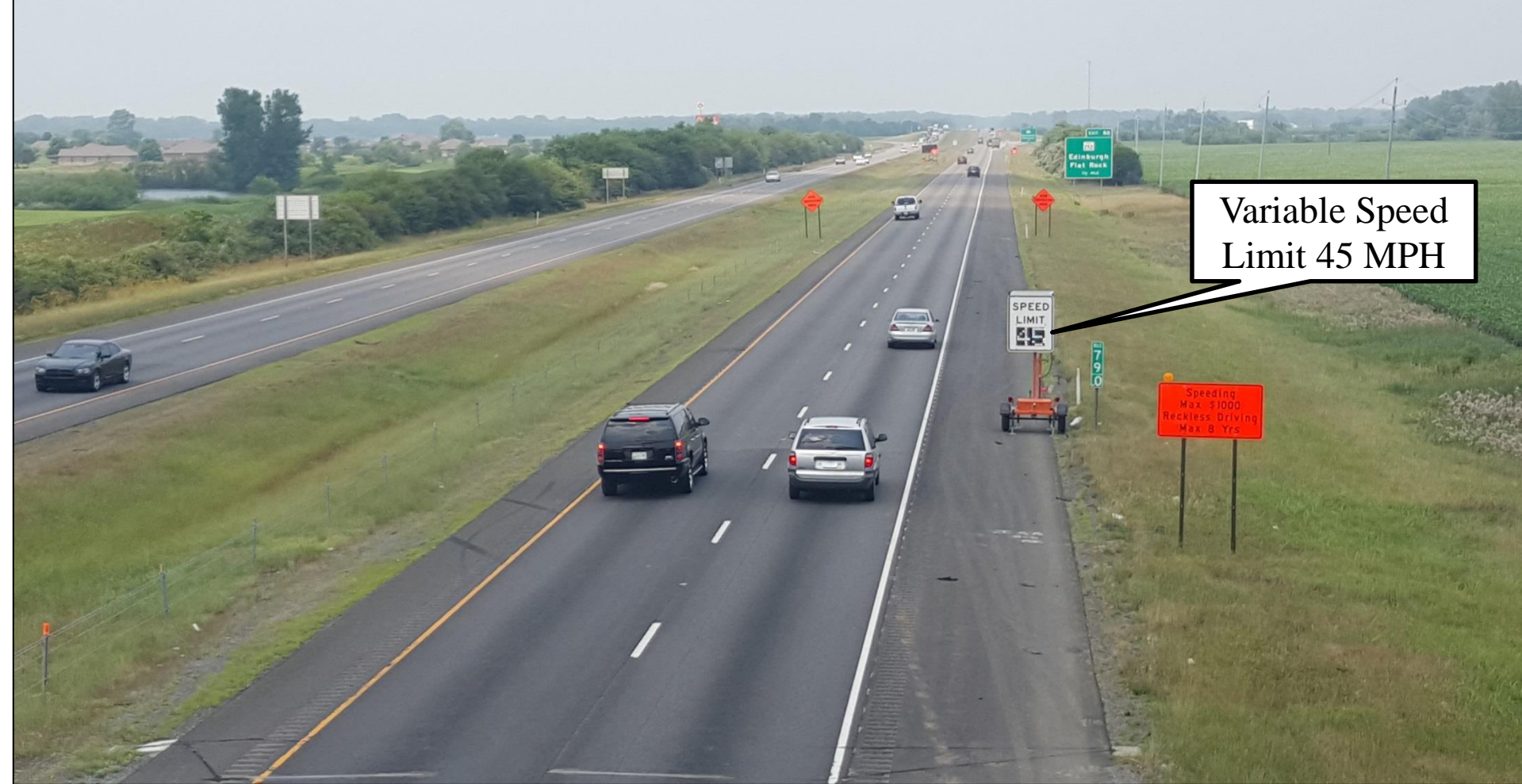
Single Variable Speed Limit Sign at I-65 NB Mile Marker 79
