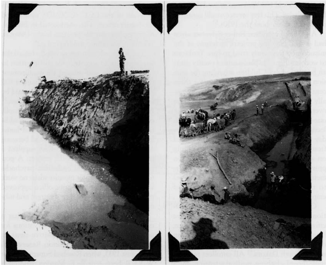
FIG. 4. (left) Problems Arise on Dam Number 75. Water and mud slowed progress and had to be removed. (right) Work on Dam Number 75. Crews and a mechanical shovel create a trench to prevent future seepage. Source: Report on Dam Number 75, Box 4, Narrative and Pictorial Reports, Records of the CCC-ID, RG 75, National Archives.
