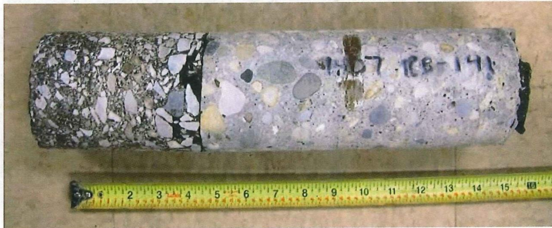
PC_S2-RB-141 – Station 278+00, Line “I65”, SB Slow Lane
