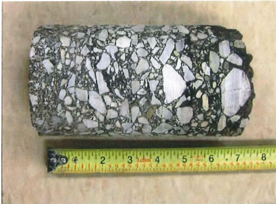
PC_S2-SB-40 – Station 298+00, Line “I65”, SB Shoulder
