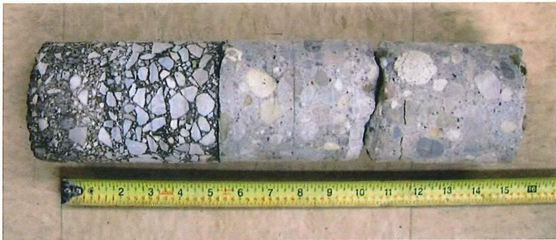
PC_S2-RB-87 – Station 170+00, Line “I65”, SB Fast Lane
