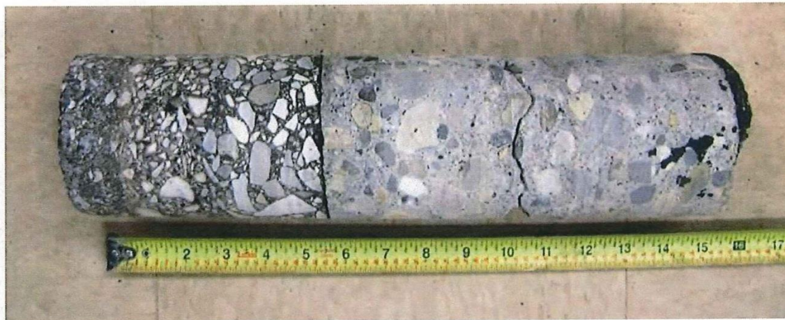
PC_S2-RB-144 – Station 290+00, Line “I65”, NB Slow Lane
