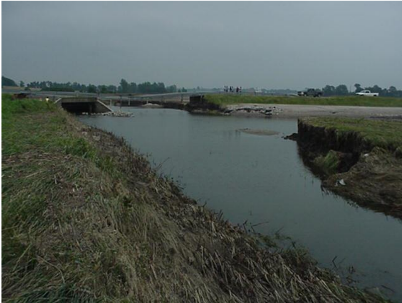
2008 site photo, view from downstream
