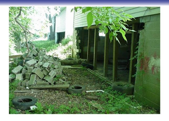
Partial clean-up of debris. Note post and beam temporary support.
