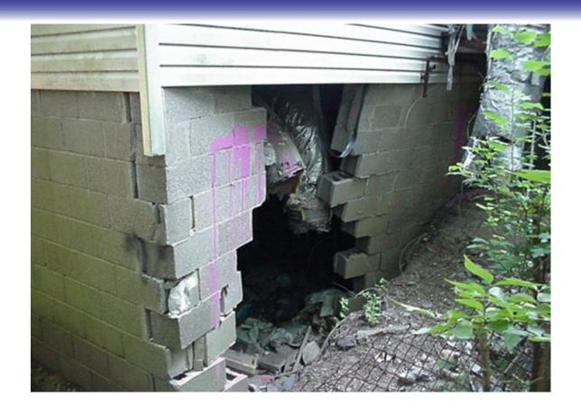
Western most structure crawlspace damage. Foundation was pushed inwards at base.
