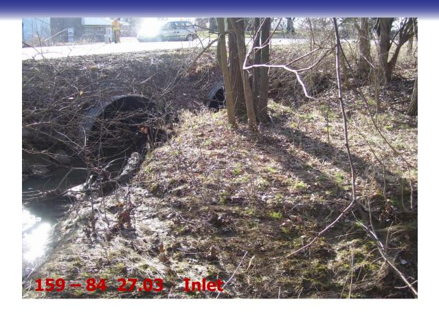
Double culvert where the stream has shifted and abandoned the other culvert, which now has a ridge of soil with trees growing immediately upstream of the inlet.
