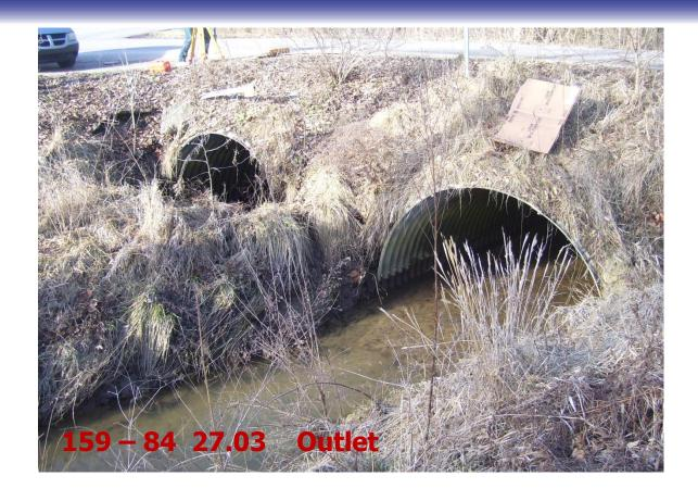
At the outlets it is apparent that the other culvert has been abandoned by the stream.
