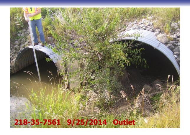
At the higher culvert outlet sediment and debris accumulation is visible, as well as a tree starting to grow.
